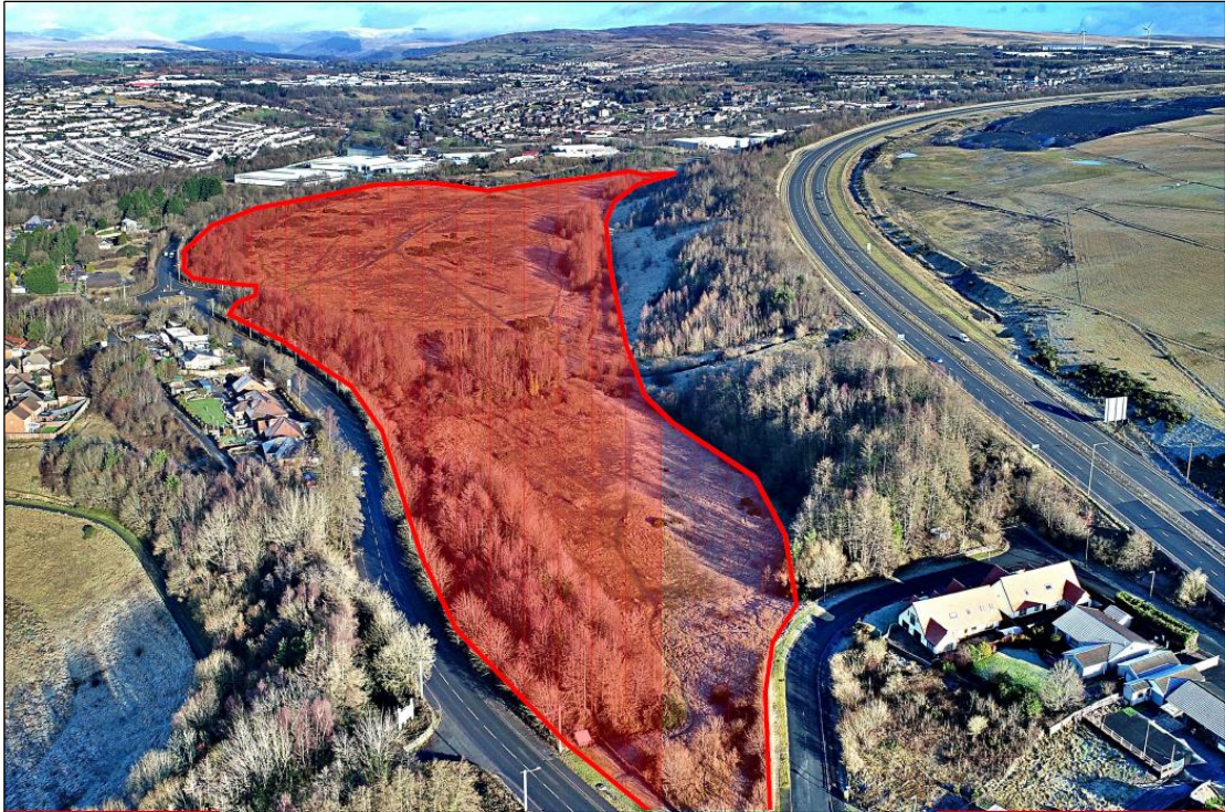
Figure 1.2: Drone aerial image of the site and surrounding area
