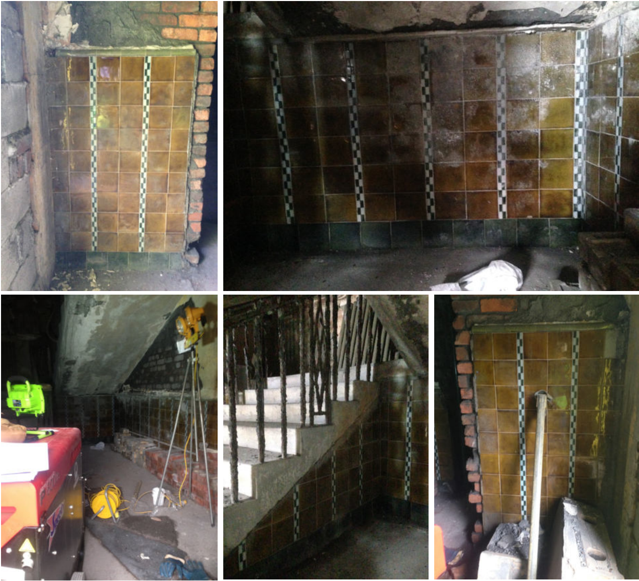
A 557.3 EXISTING CONDITION SITE PHOTOGRAPHS
