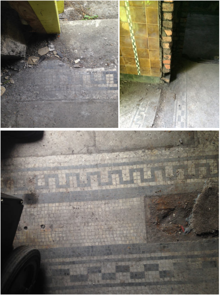
A 557.8 EXISTING CONDITION SITE PHOTOGRAPHS
