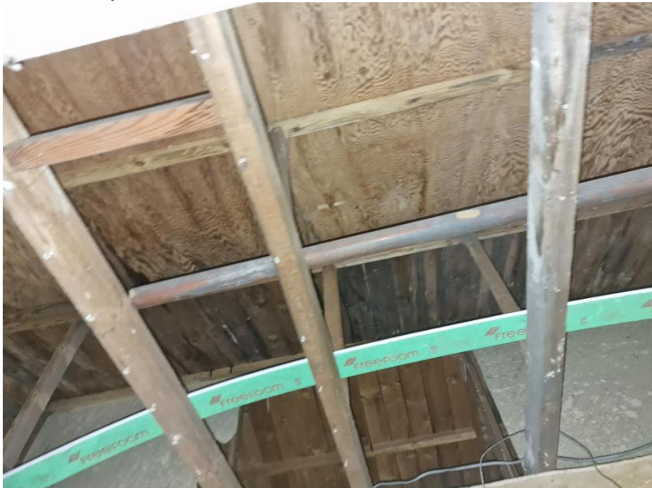
Plate 2- example of underside of cabin roof
