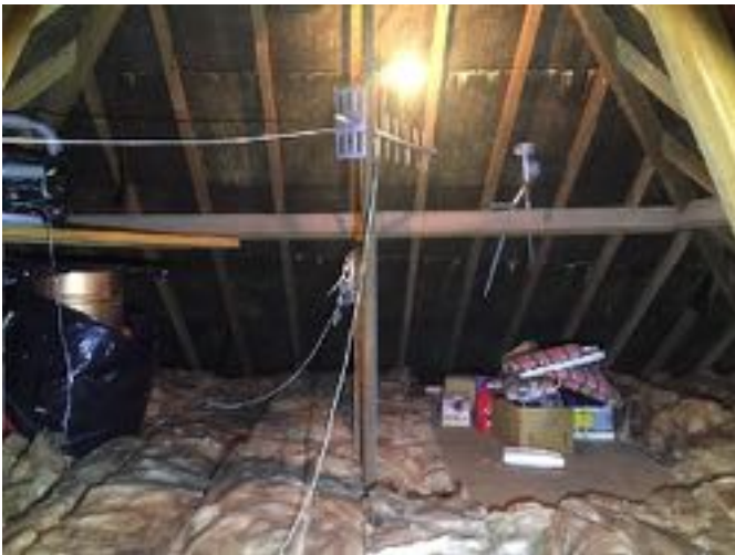
View of attic space
