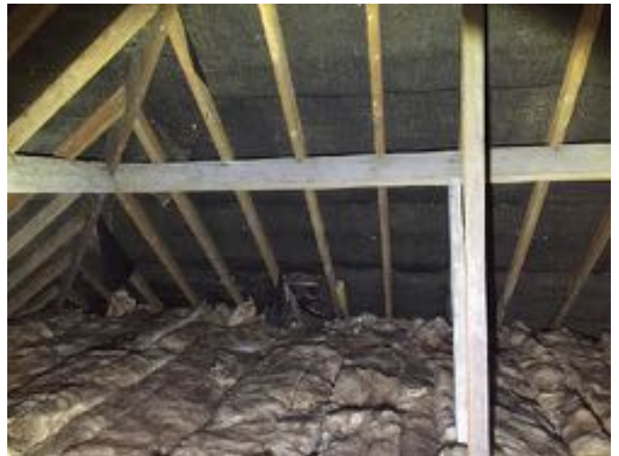
View of attic space
