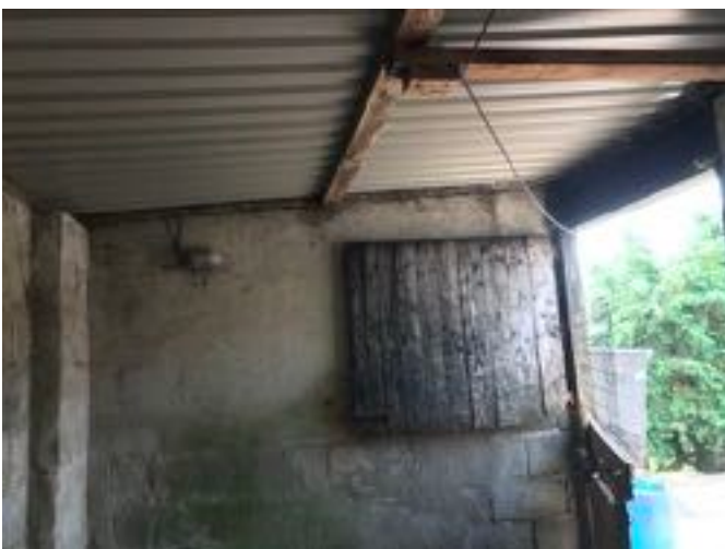
Internal view of outbuilding
