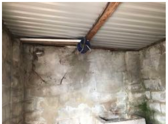
Internal view of outbuilding
