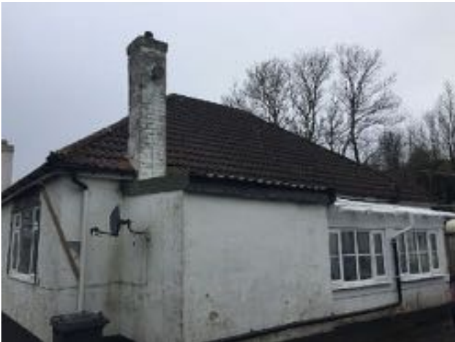
Eastern (rear) elevation of the building
