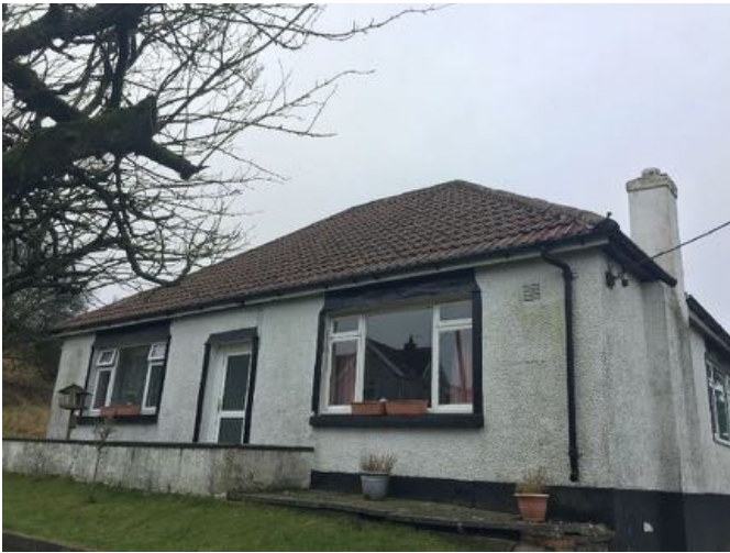
Western (front) elevation of building
