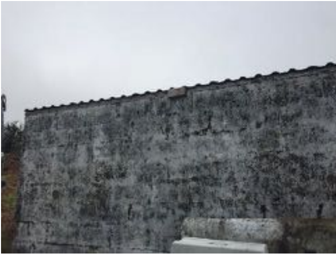
View of outbuilding roof line
