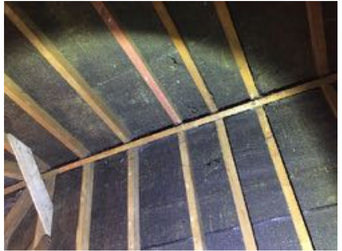
View of ridge board in attic space
