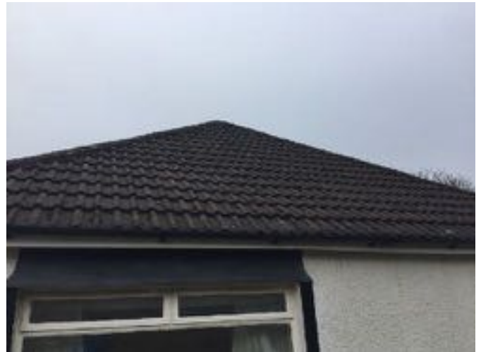
Northern elevation of building
