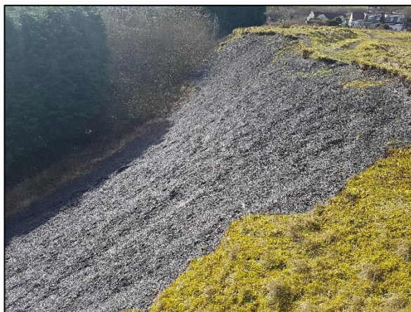
Photo 10: Exposed colliery spoil
