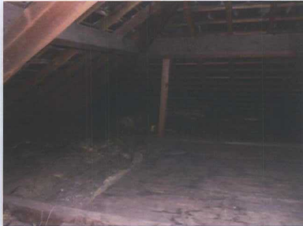
Figure 7: Roof void within residential dwelling
