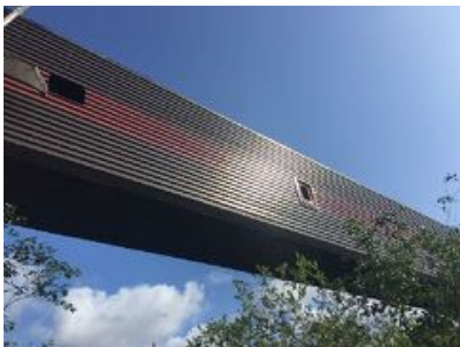
View of gantry over River Taff
