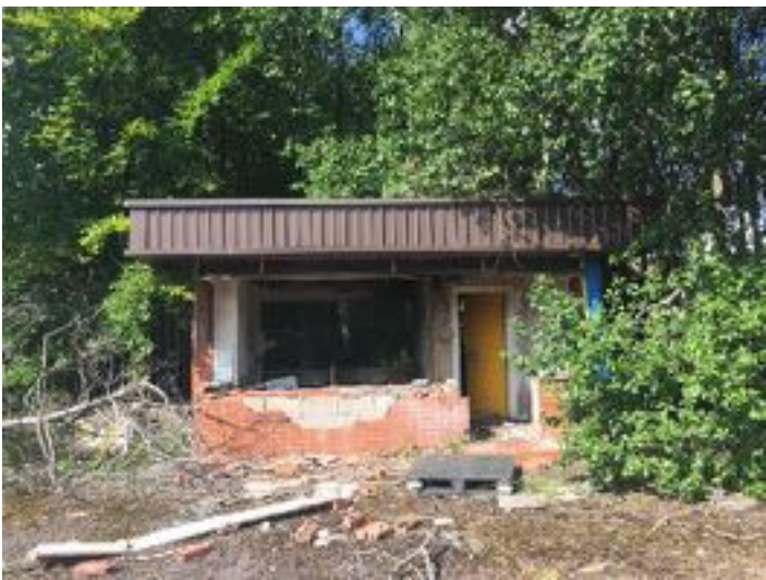
Remaining small building
