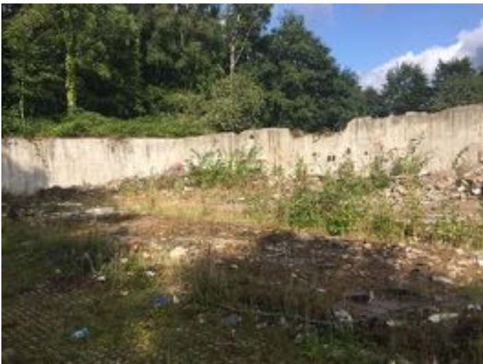
View of building foundations
