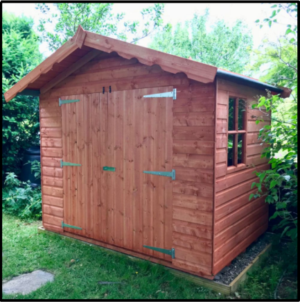
New garden shed to be traditional horizontal shiplapped timber proprietary unit with double access door and window, shed size to be 2100 x 1800 x 2300mm approx.
