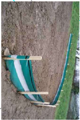
TYPICAL SILT FENCE CONSTRUCTION
