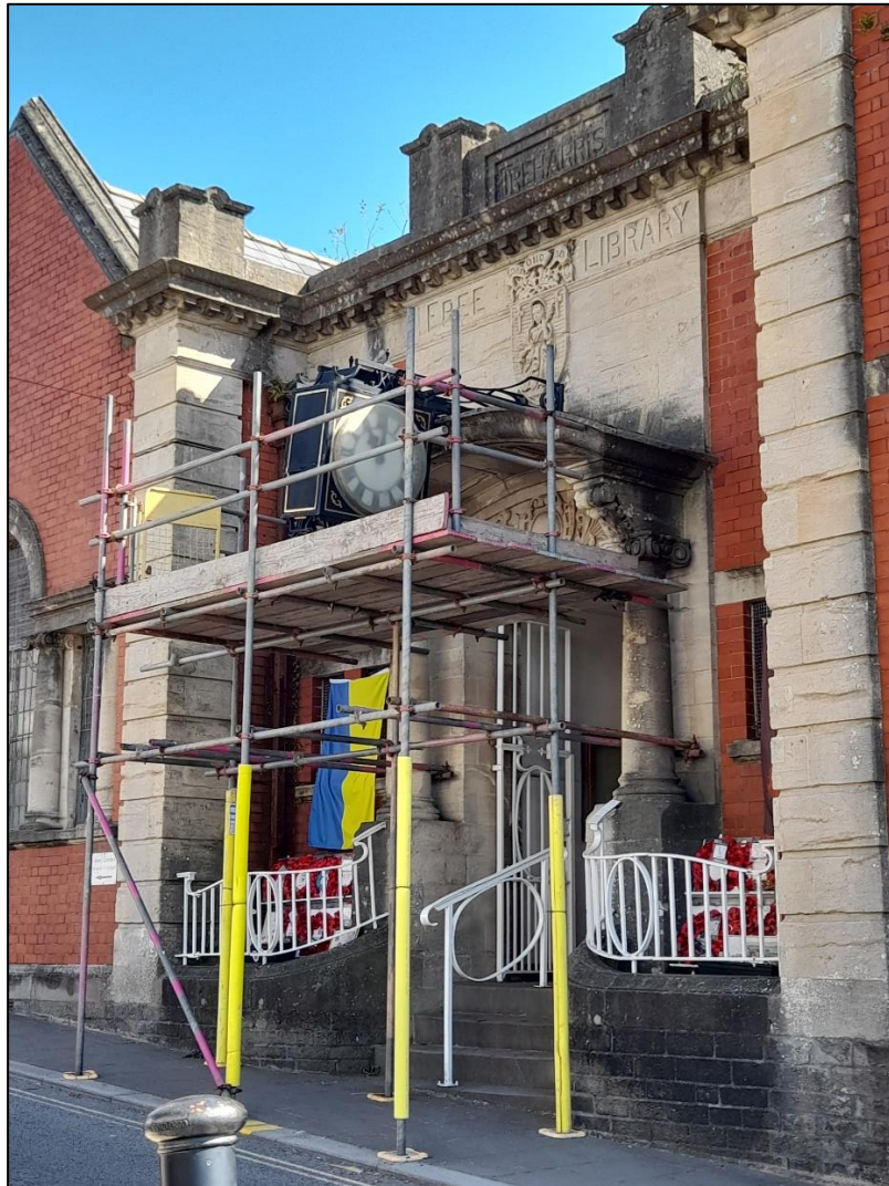
Plate 5. Main entrance including memorial clock, looking north-east.
