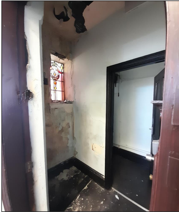
Plate 21. Cloakroom and toilet in south-west of library, looking north-west.
