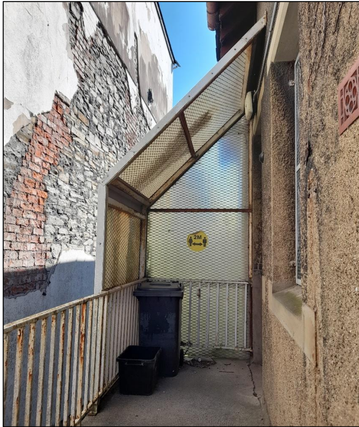
Plate 7. Canopy over door on north-facing elevation, looking east.
