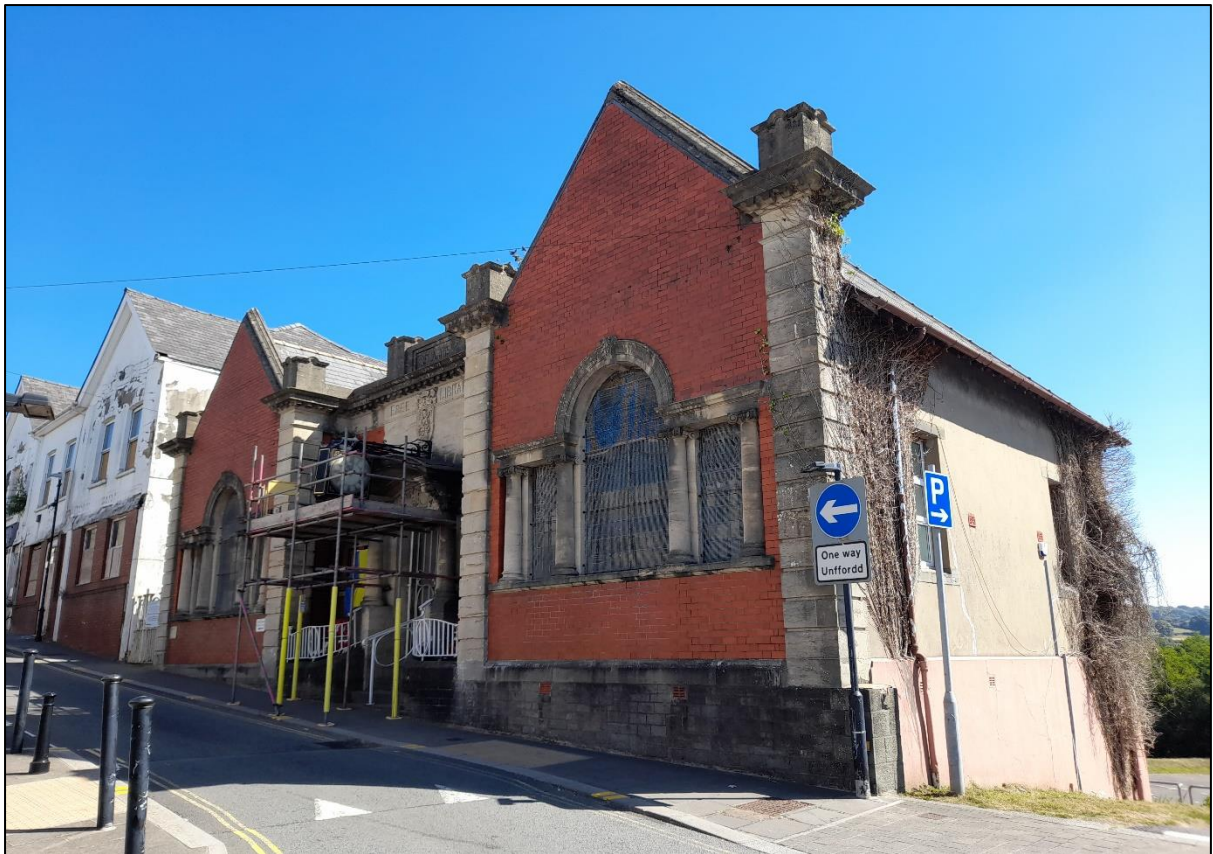
Plate 1: Front elevation of Treharris Public Library, looking north-east.
