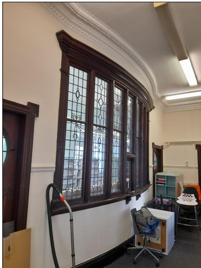
Plate 10. Reception window, looking south.
