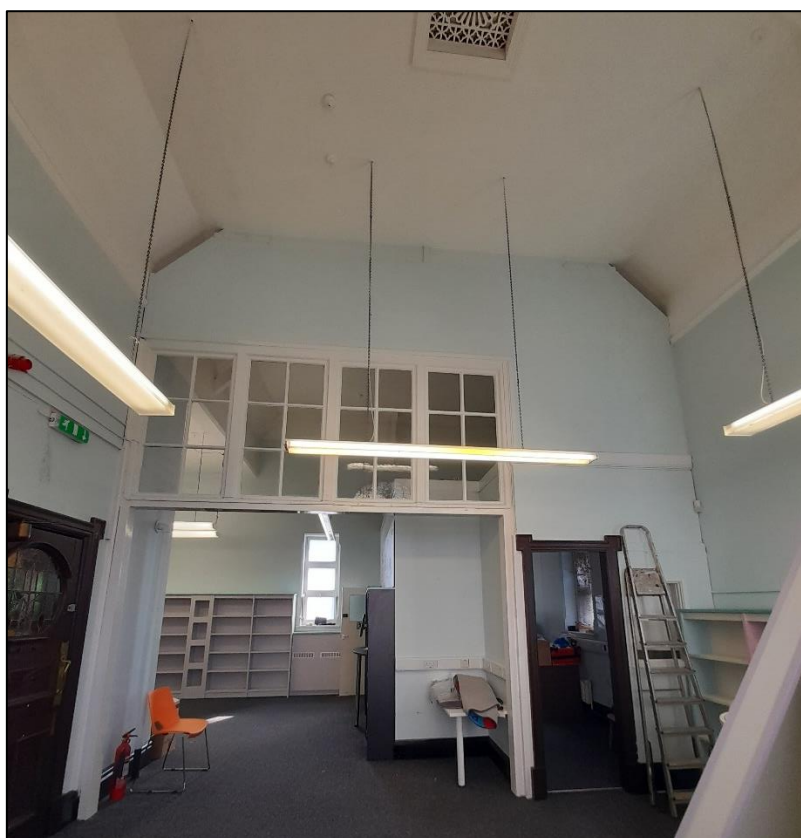
Plate 12. South end of main library room, looking east.
