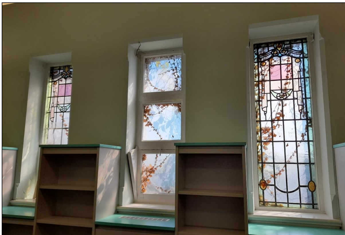
Plate 14. Windows on the centre of the east wall of the library, central window is a later replacement.
