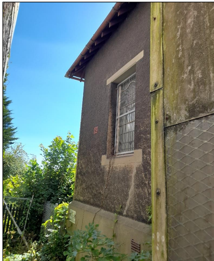
Plate 8. Window to east end of north-facing elevation, looking south-east.
