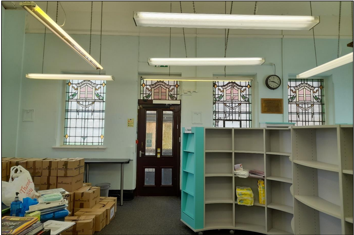
Plate 15. North-wall of library with side door.
