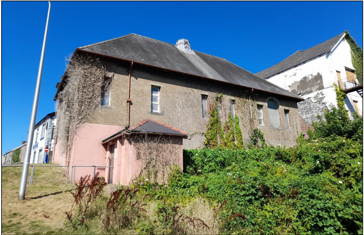
Plate 3. East-facing elevation of Treharris Public Library with single storey rear extension. Looking north-west.
