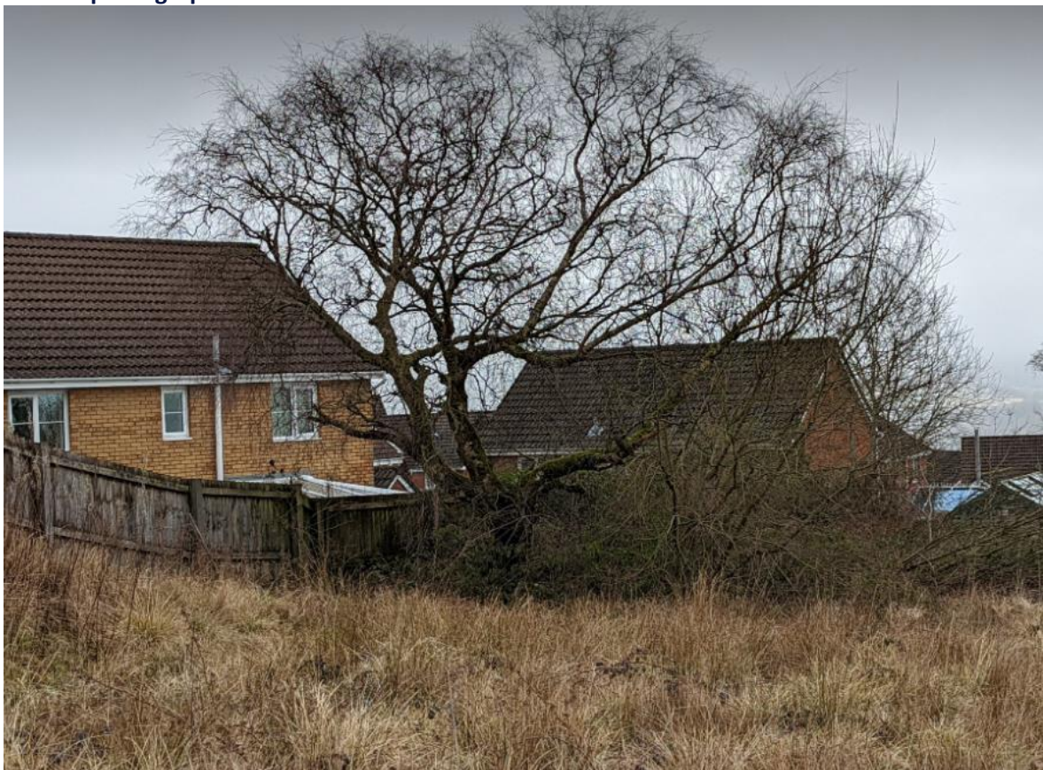
Plate 6- photograph of tree to be removed
