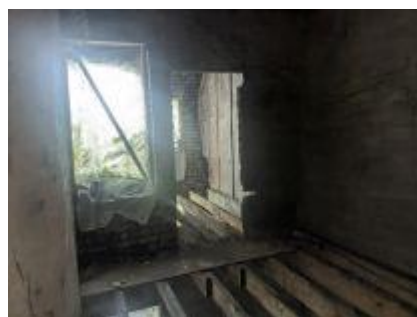
Plate 8 – First floor – roost entrance from the interior.
