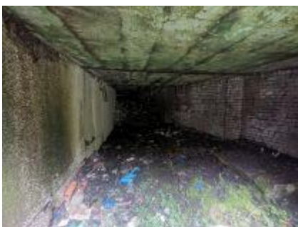
Plate 5 – Taken at the entrance of Building B – from the central courtyard, facing east.
