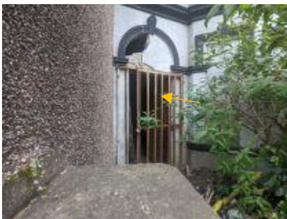
Plate 3 – Gated doorway at the main service road providing access to the interior.
