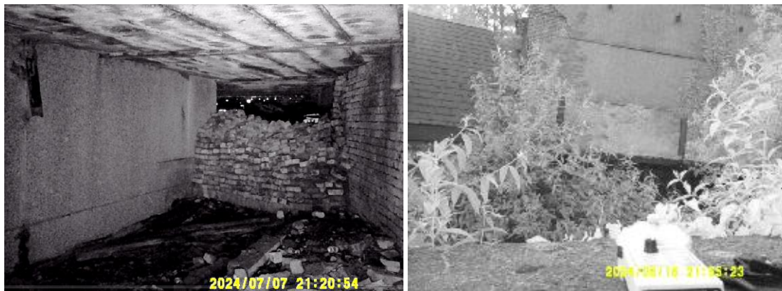
Plates A & B: Infrared Monitoring (Image quality): showing the interior of Building B and the Rear of the property. Locations are identified in Appendix D.
