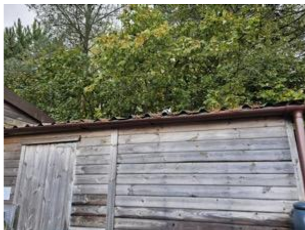
Photo 9: Roof at the North-Western Elevation
