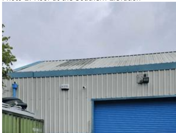
Photo 2: Roof at the Southern Elevation
