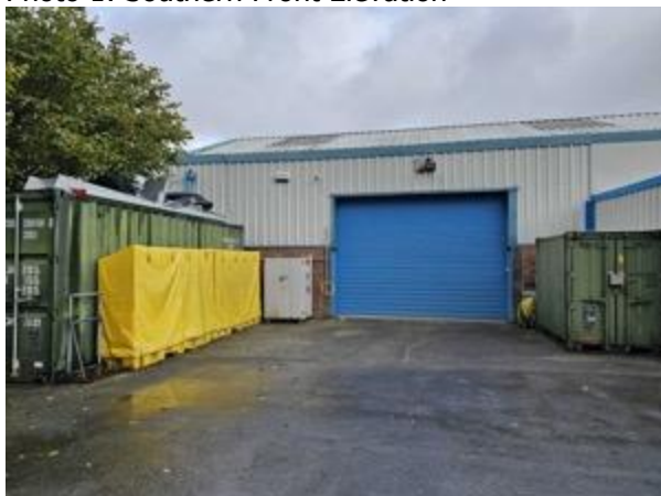
Photo 1: Southern Front Elevation
