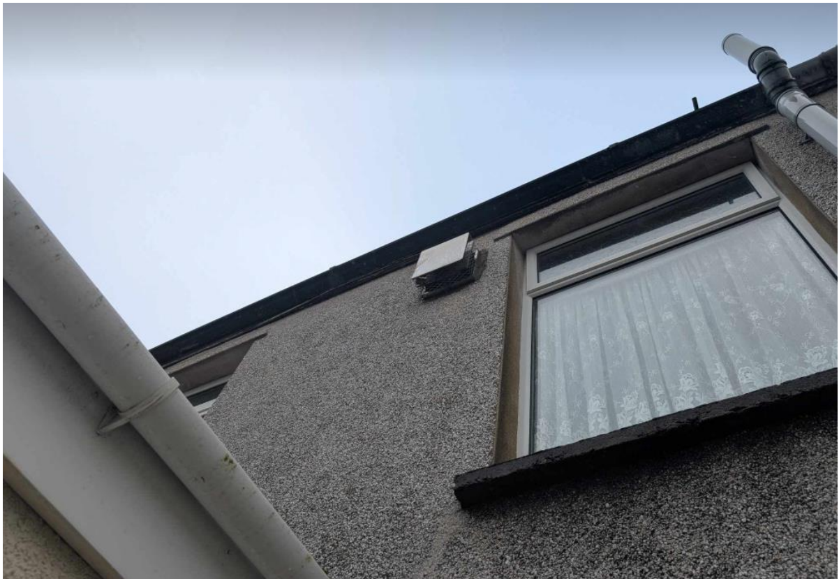
Plate 6- Photograph of gap beneath rear fascia board
