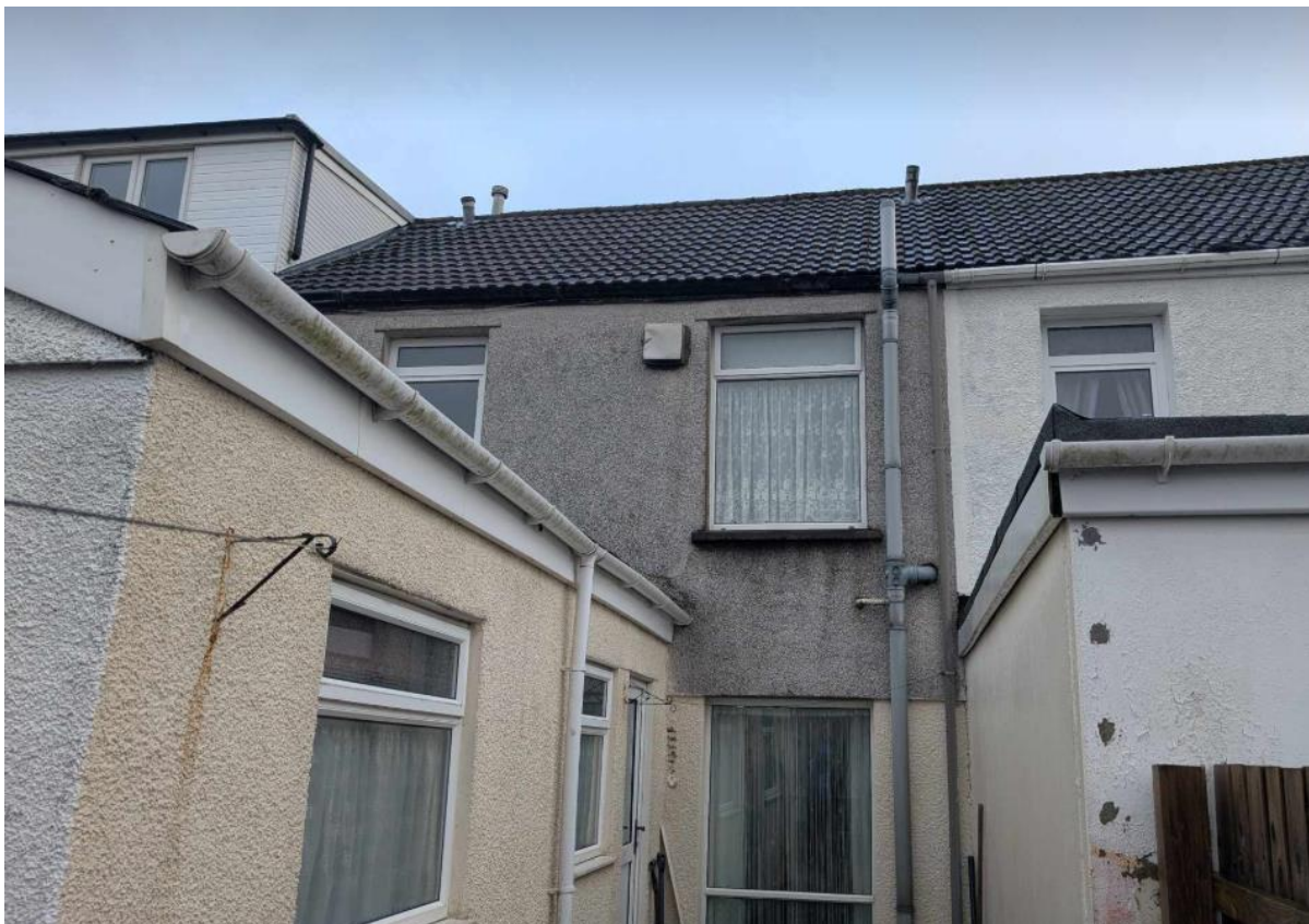
Plate 8- photograph of rear roof
