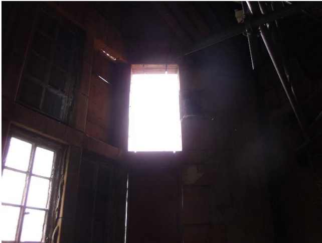
Figure 10: Broken window on top floor of building allow bird and bat access
