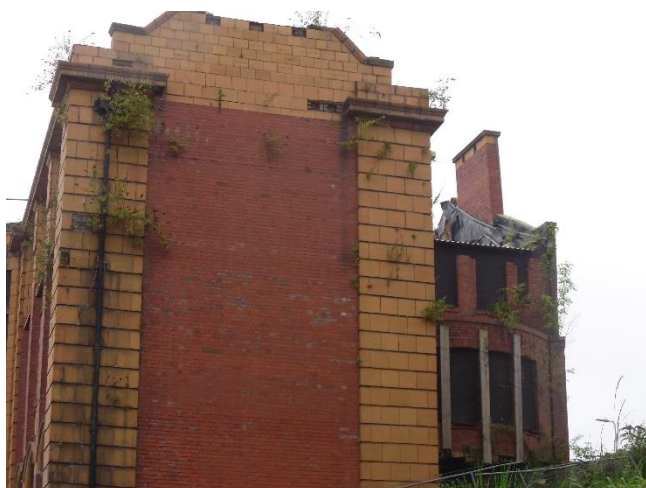
Figure 16 - Eastern aspect of building
