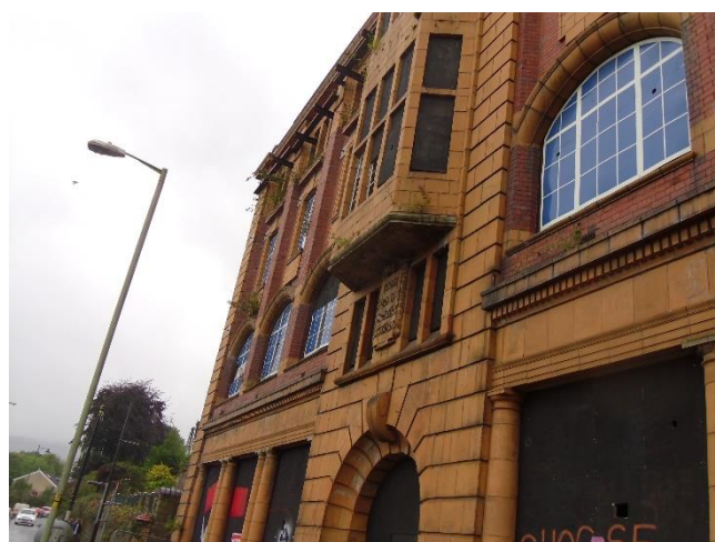
Figure 17 - Front of building
