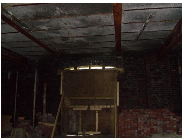
Figure 8 - Upper floor at the rear of the building (internal image)
