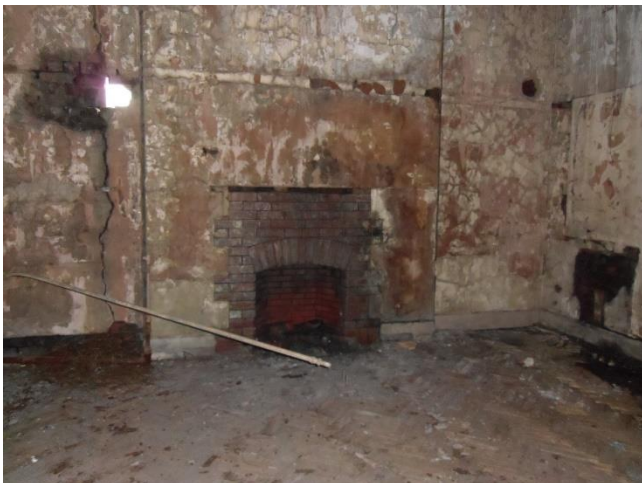
Figure 14 - Fireplace on the second floor of building
