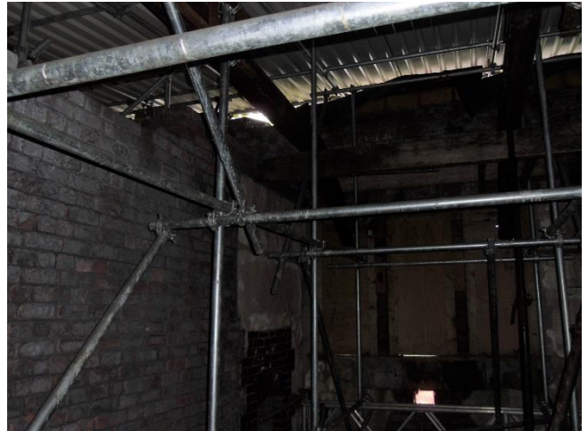
Figure 11 - Temporary roof to the rear of the building
