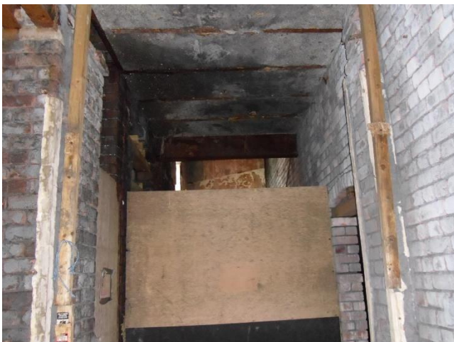
Figure 6 - North eastern corner of the building (Internal), location of where lesser horseshoe bat entered the building, blocking off human access into lift shaft.
