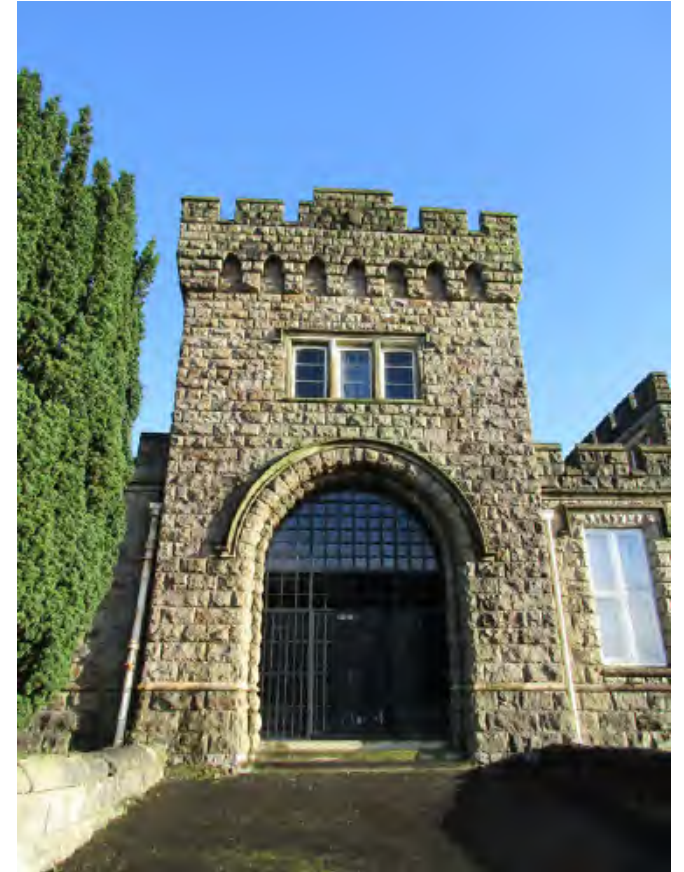
West gatehouse (former Stable entrance)
