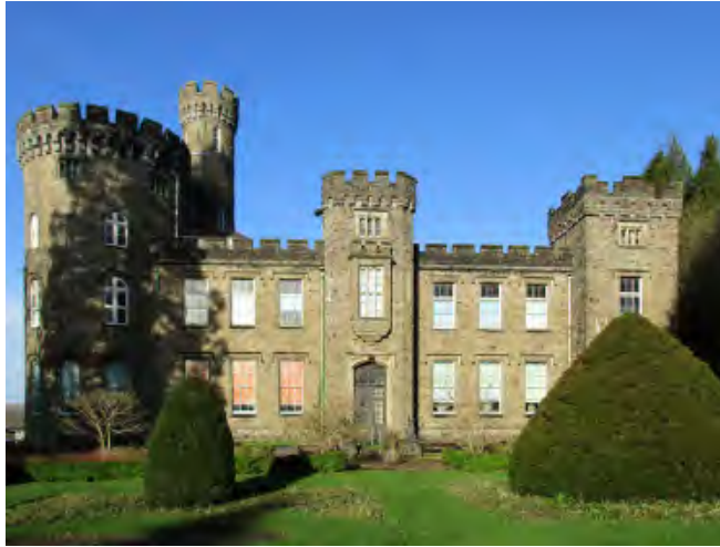
East elevation and former family entrance
