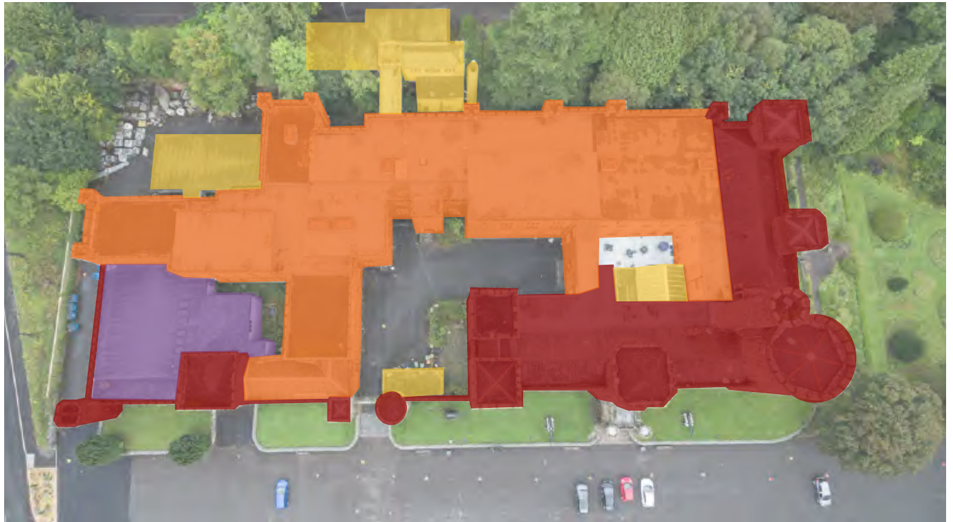
Image captured in a drone survey of the Castle circa 2016, annotated to show the relative age of the built fabric.
