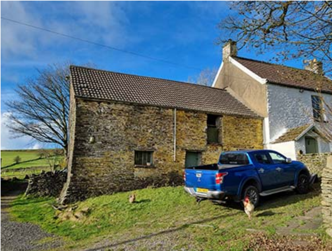
Photo of front elevation of barn showing it attached to main farm house
