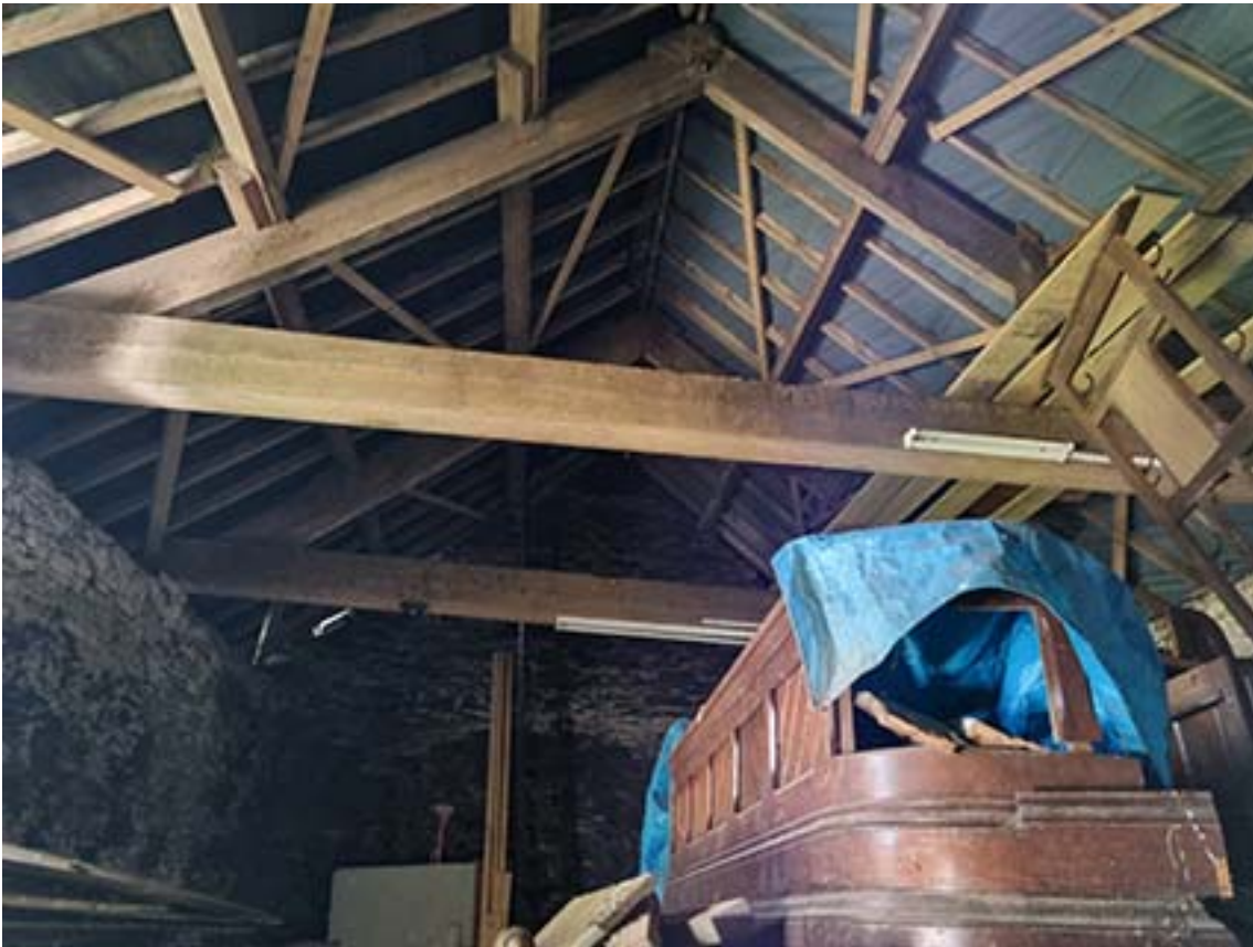
Photo of showing cut roof trusses, purlins and rafters with more recent diagonal bracing
