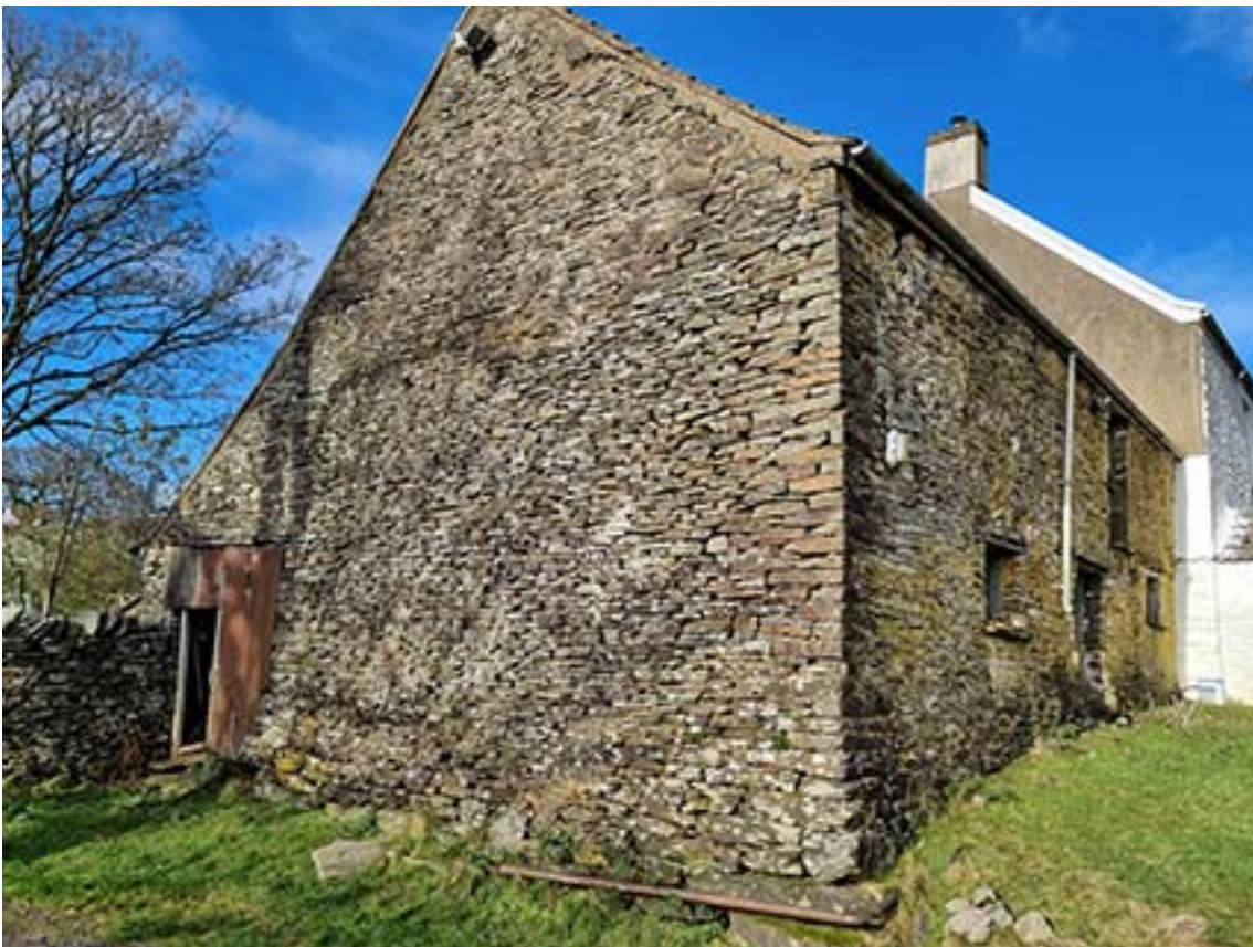
Photo of gable elevation showing lower external ground levels
