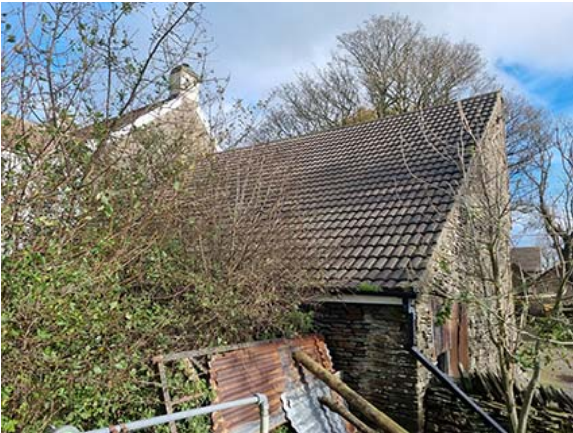
Photo of rear roof of barn extending over rear out-buildings
