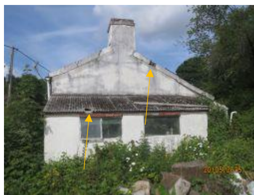
Exterior – Eastern elevation - multiple PRFs recorded.
