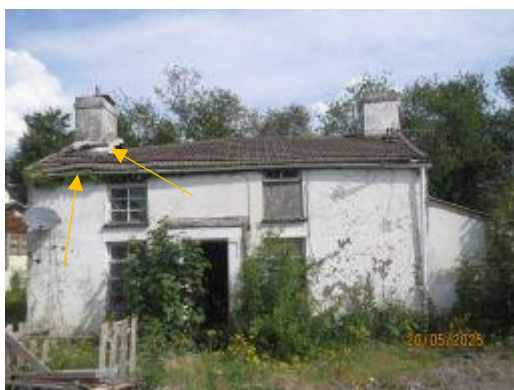
Exterior – Southern elevation - multiple PRFs recorded.
