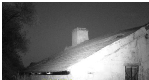
Plate A: Infrared Monitoring (NVA - Image quality)
