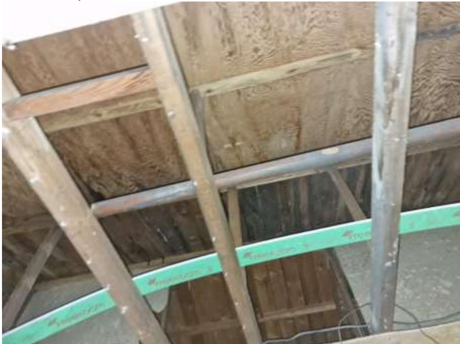
Plate 2- example of underside of cabin roof
