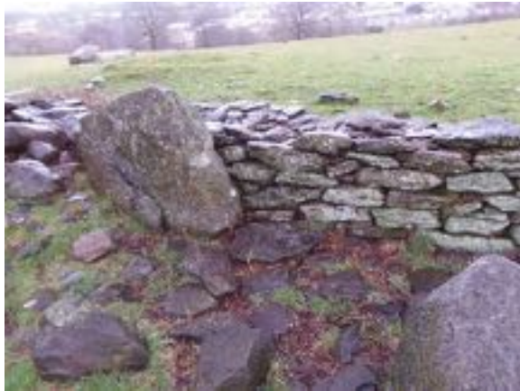
Pile of stones where dry stone wall has collapsed, eastern boundary
