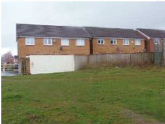
Section of western boundary of breeze block
