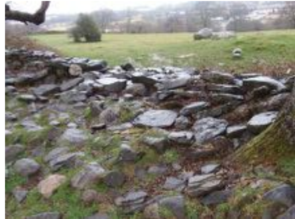
Pile of stones where dry stone wall has collapsed, eastern boundary
