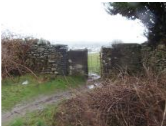
Access to field in south east corner
