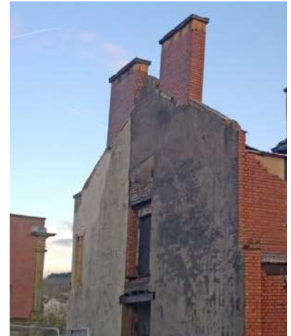
The existing rear elevation of the Middle Building.
