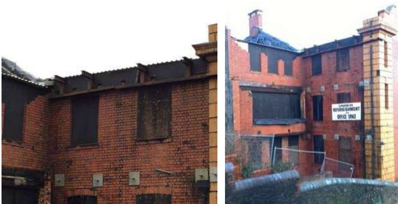
Above: The location of the 'penthouse' dormer proposed within the recreated 'Rifle Range', the original historic fabric being entirely missing. Note also the condition of the original curved oriel windows, new steel 'props' being introduced to provide required support beneath.
