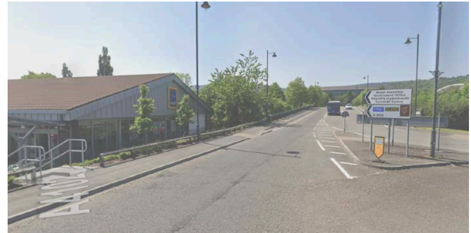
View from roundabout showing level difference from Aldi store to A4102 leading onto bridge.
