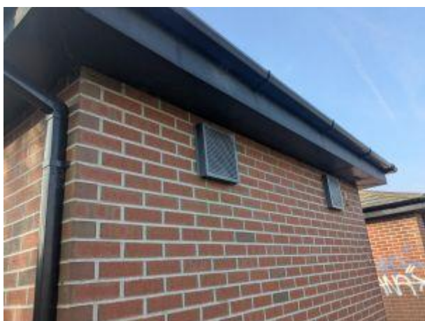
No PRFs – Sealed soffits and bargeboards.
