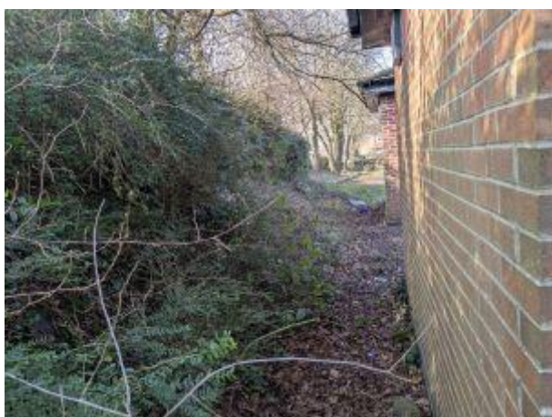
Southern elevation adjacent to hedgerow (introduced shrub).
