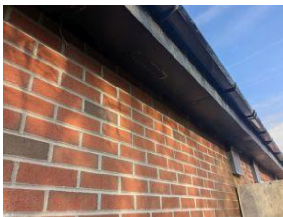
No PRFs – Sealed soffits and bargeboards.
