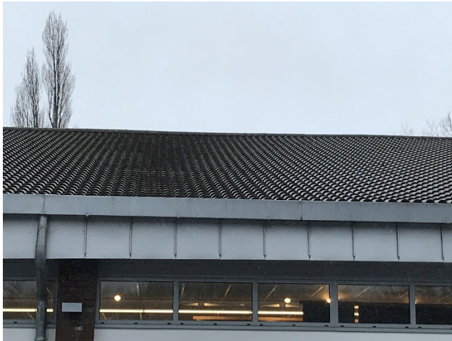
Photograph 2: Tiles on the roof of B1 are in good condition.
