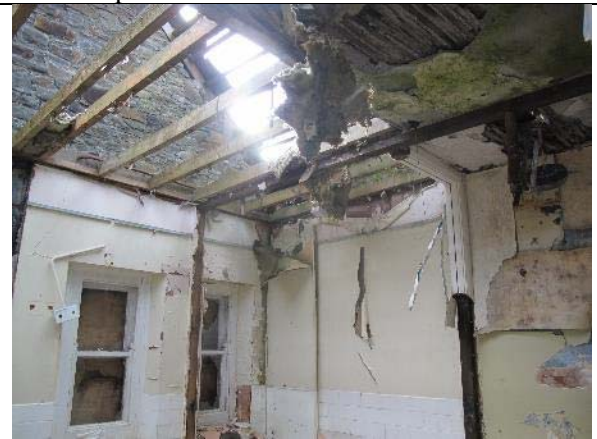
Interior of building 1
