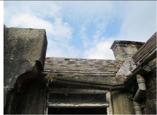
View of part of western elevation
