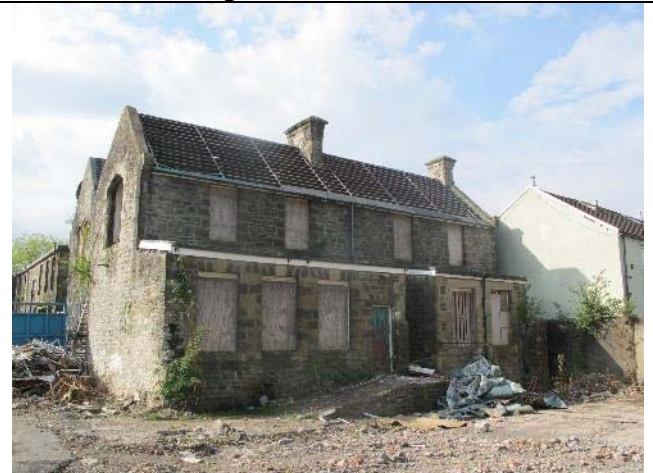
Northern elevation of building 1
