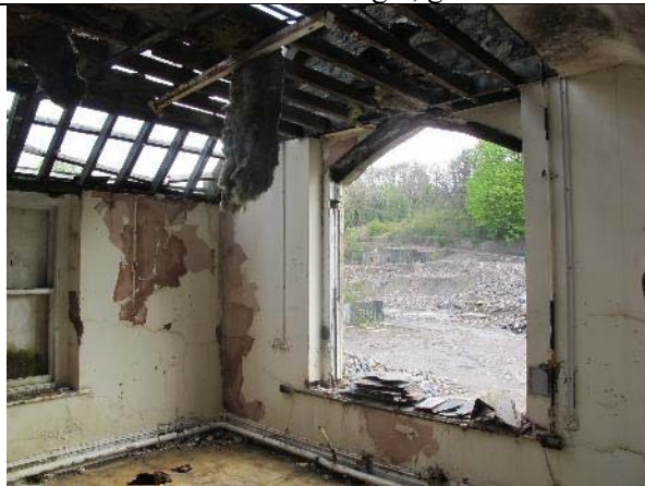
Large open window on the western elevation
