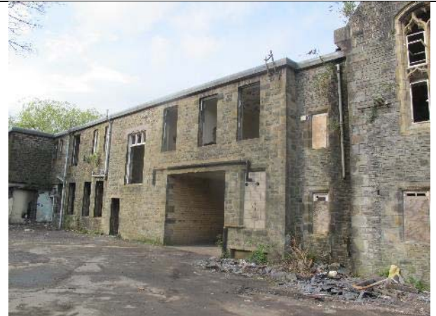
Western elevation of building 1
