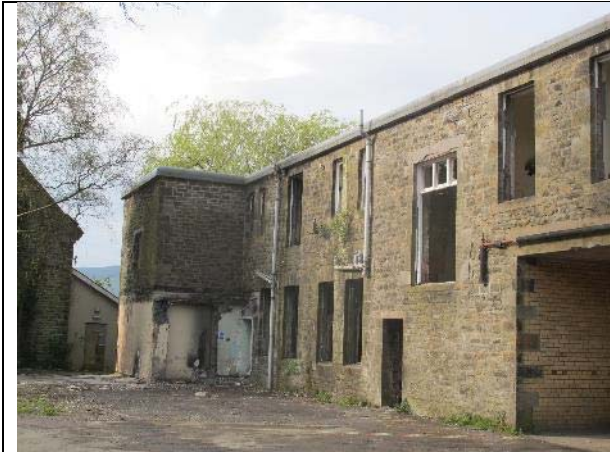
Western elevation of building 1
