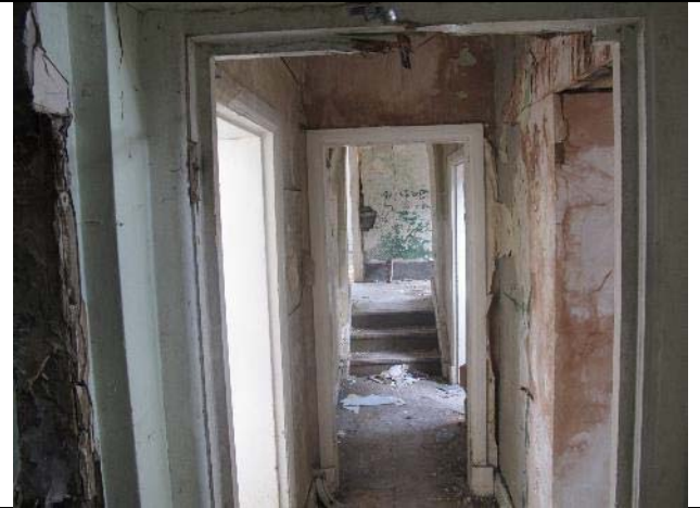
Interior of building 1
