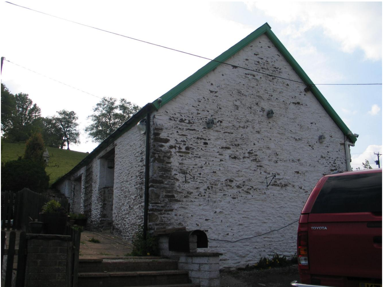
East gable and south elevation
