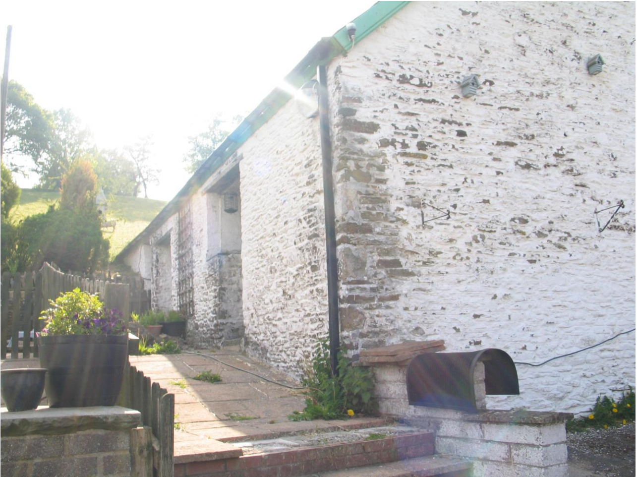
South elevation and south corner of west gable
