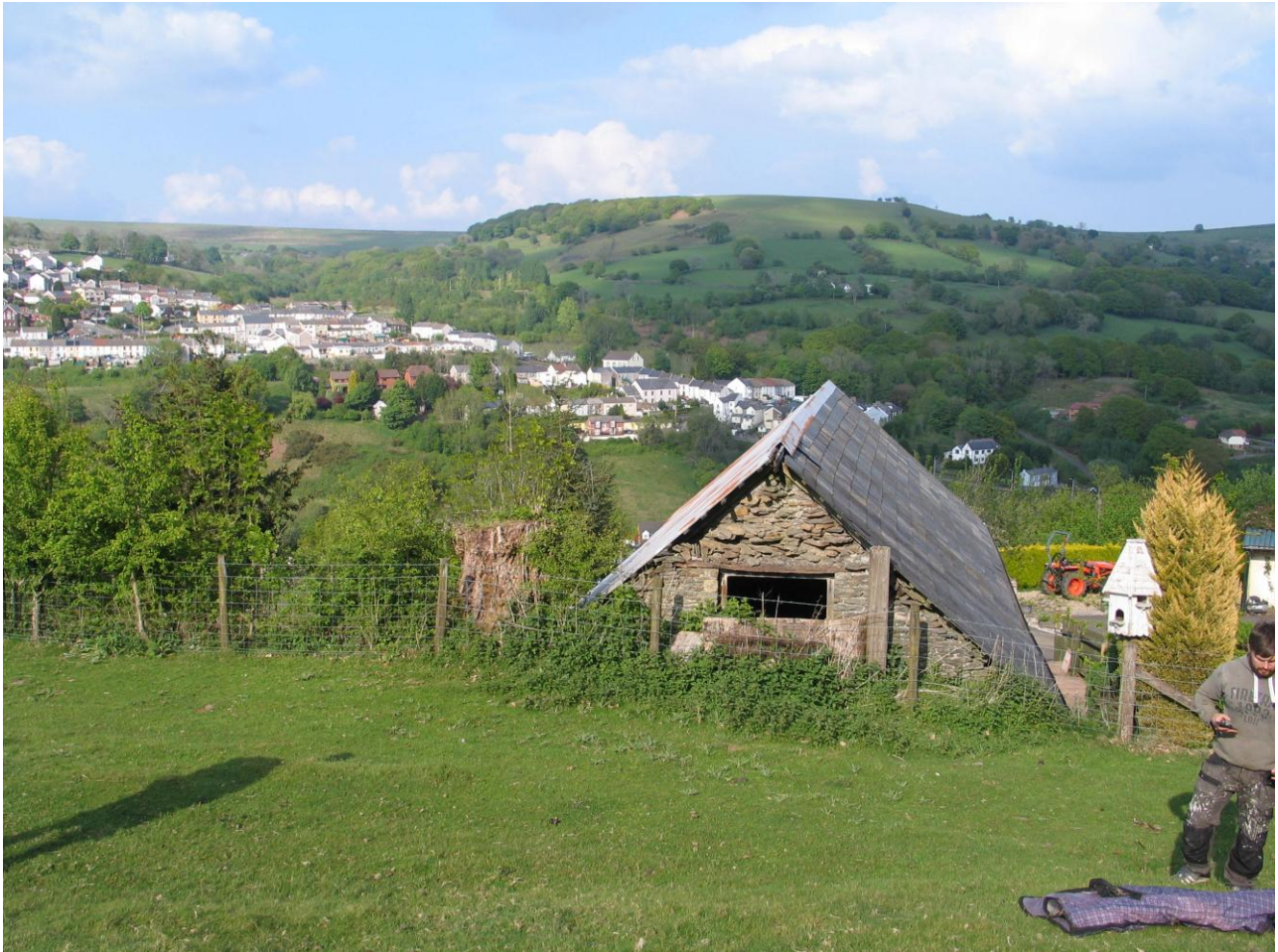
Roof covering, metal sheets to north slope and slate to south slope
