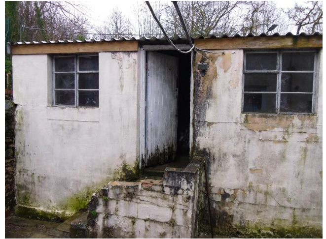
Figure 8 - Garage (door is closed and locked when not in use)
