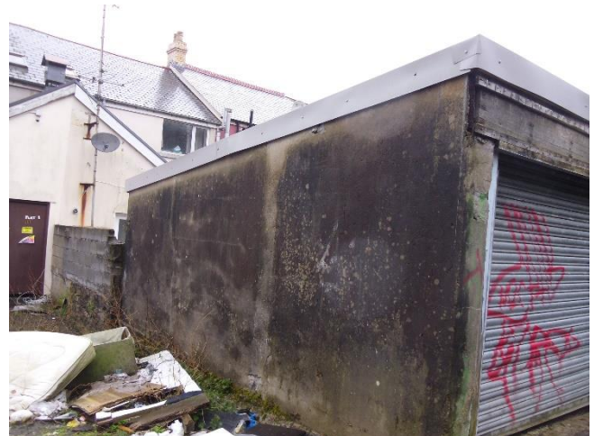
Figure 6 - Western aspect of the garage and roof of terraced property
