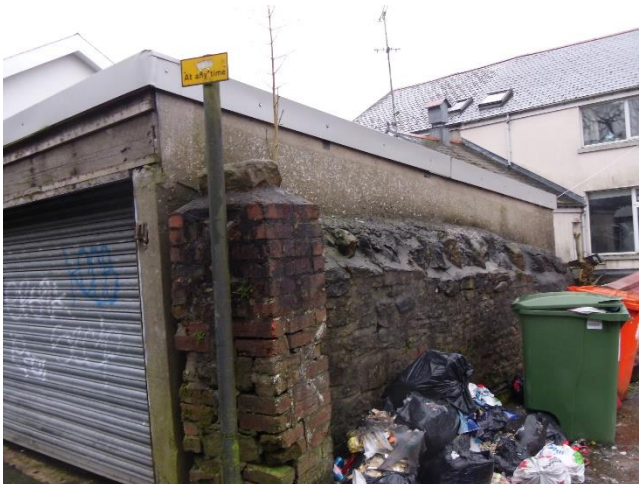
Figure 5 - Eastern aspect of garage and roof of terraced house
