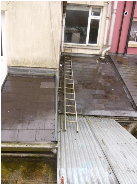
Figure 3 - Rear of terraced property
