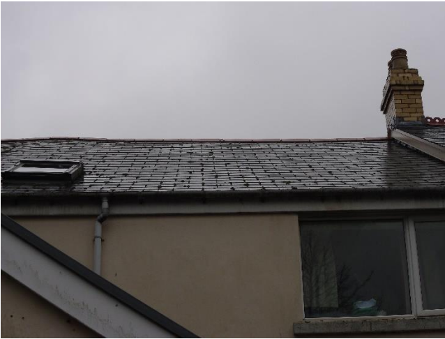
Figure 7 - Roof of terraced house
