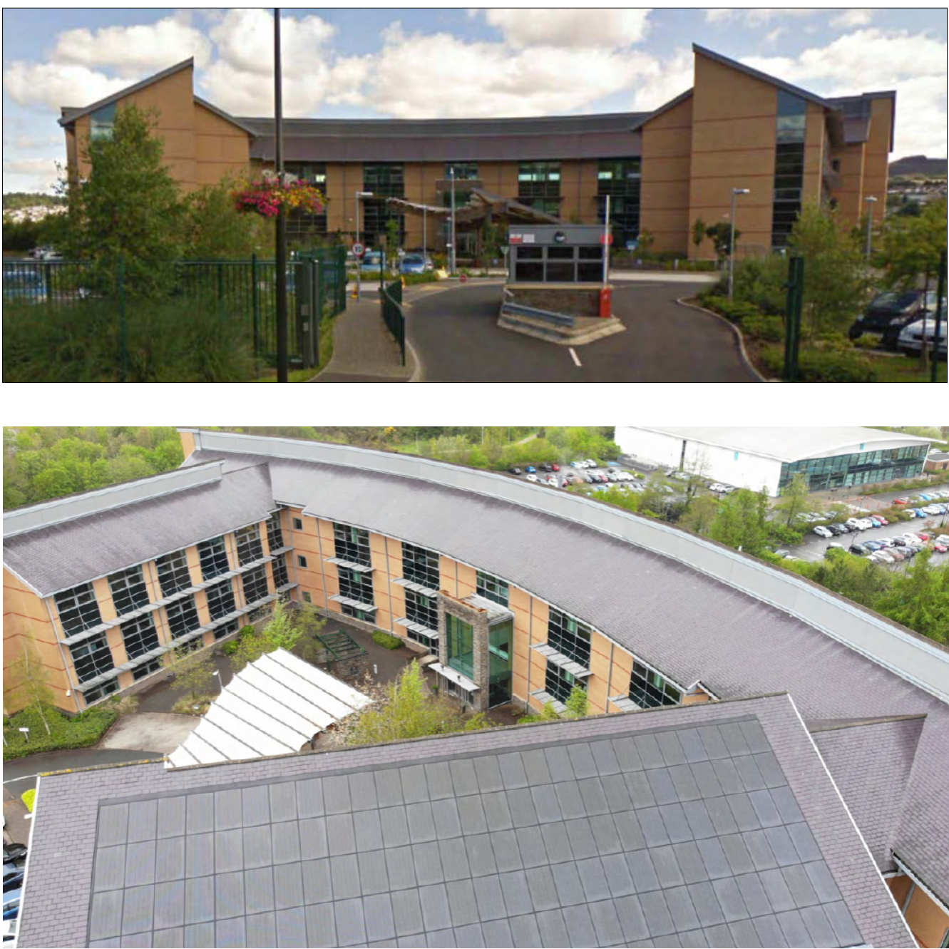
EXISTING BUILDING PHOTOS
