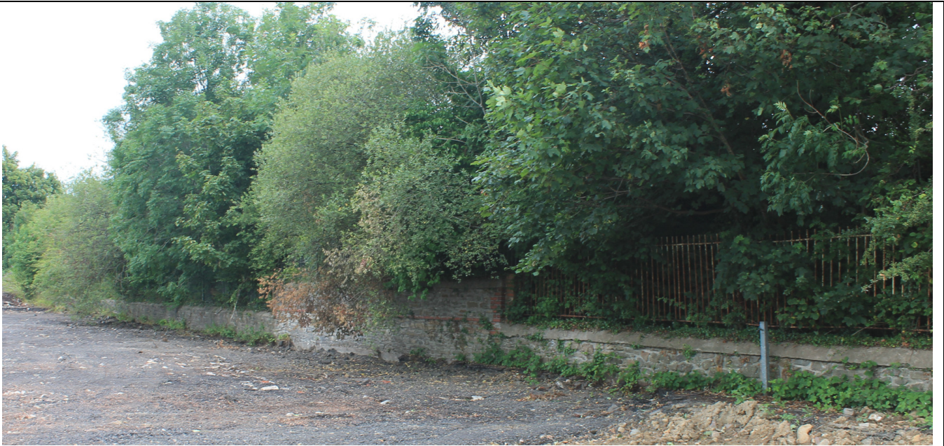
East boundary showing tree screen outside the site and the stone retaining wall
