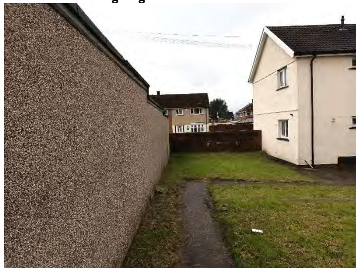
Plate 2-Communal garden to the rear of the garages.
