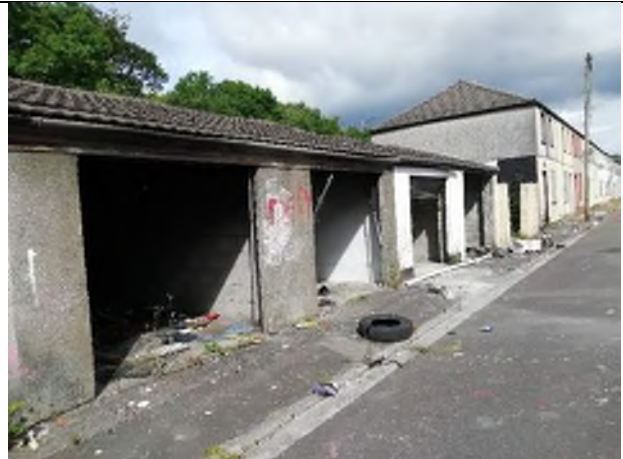
Figure 9 – Garages on Taff Street
