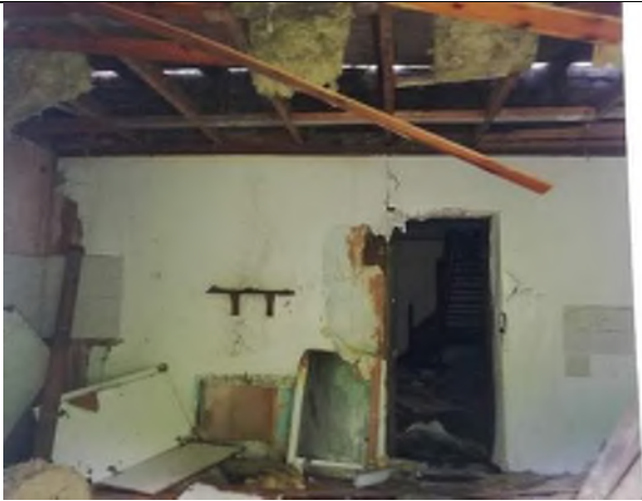
Figure 12 – Interior view (from outside) of south-westernmost property
