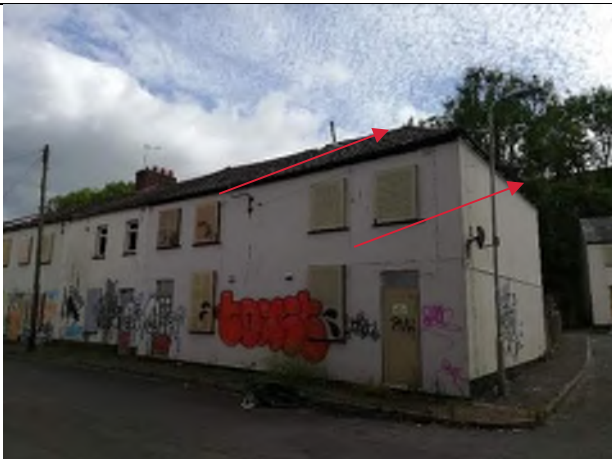
Figure 16 – South-eastern end of Crescent Street – roosts marked with arrows
