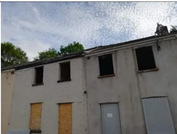
Figure 14 – View of open windows along Taff Street
