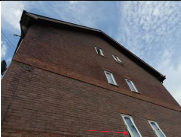
Figure 18 – Northern gable of block of flats. Partially open window (arrow) indicated entry point for single pipistrelle
