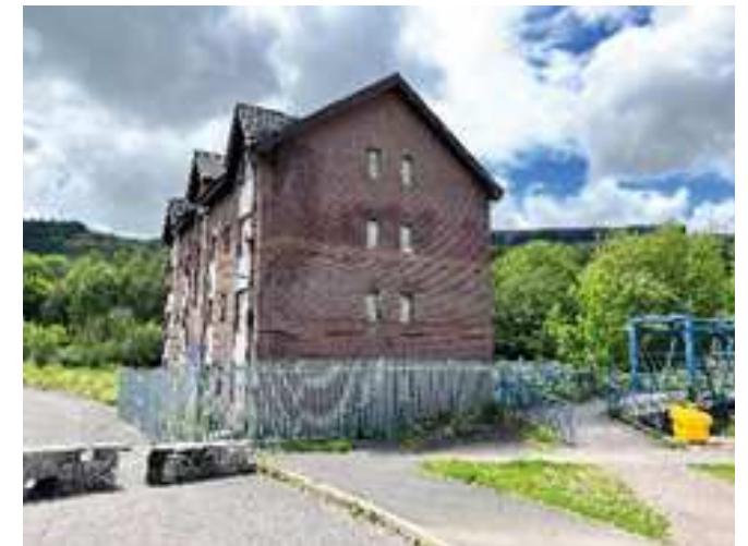
Figure 17_Site photographs of the Rechabite Hall in context
