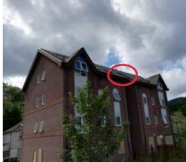
Figure 3 - Block of flats, rear aspect with soprano maternity roost identified in 2019 emergence surveys circled.
