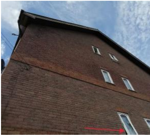
Figure 2 - Northern gable of block of flats. Partially open window (arrow) indicated entry point for single pipistrelle during 2019 emergence surveys.
