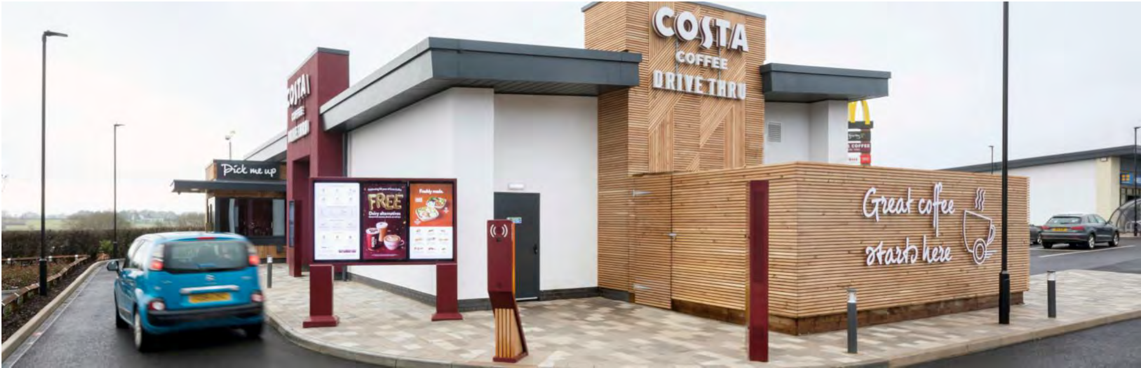
Costa Drive Thru Building & External Finishes
