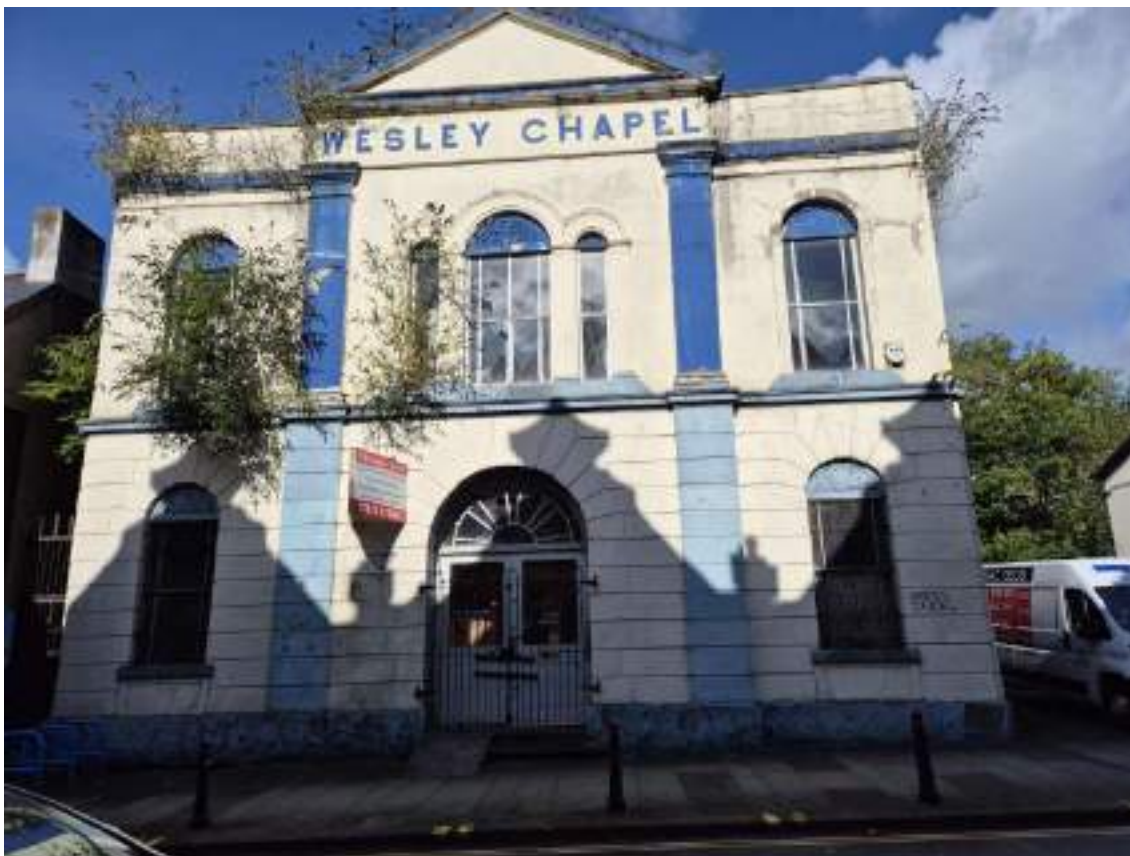
Figure 23 – Photograph of Former Wesley Chapel
