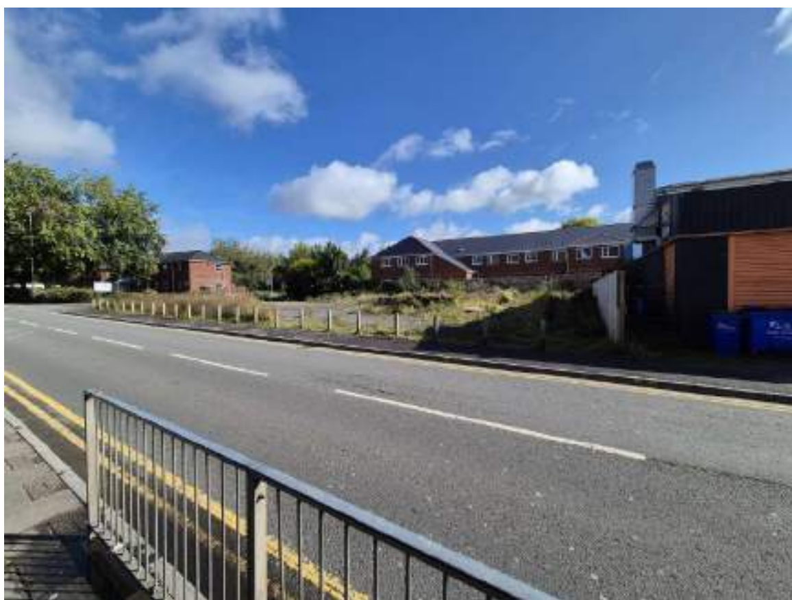
Figure 21 – Photograph of site at Dynevor Street
