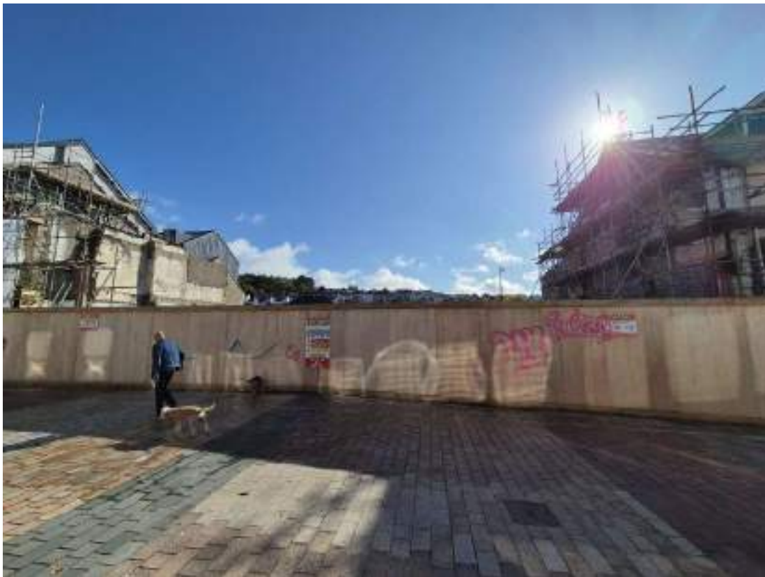
Figure 24 – Photograph of 34-38 High Street
