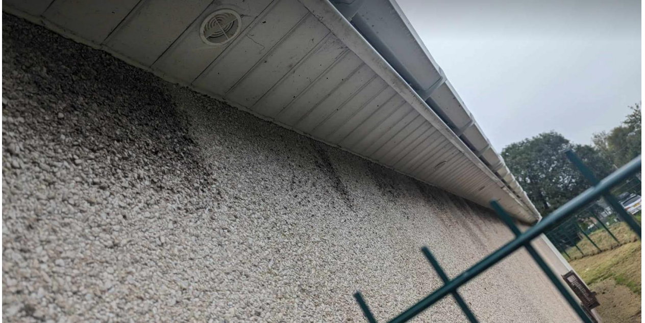
Plate 7- photograph of sealed fascias
