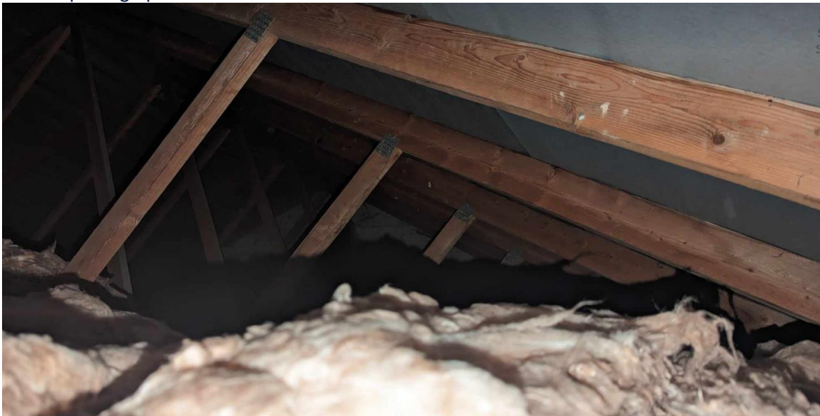
Plate 4- photograph of north western roof void
