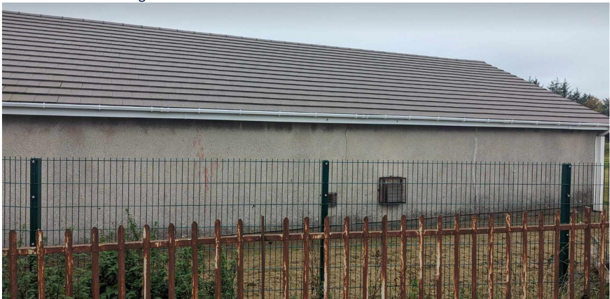
Plate 8- rear of building
