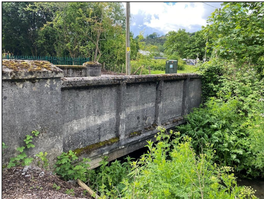
Photograph 8: Maestaf Street Bridge, photographed from the northern side.
