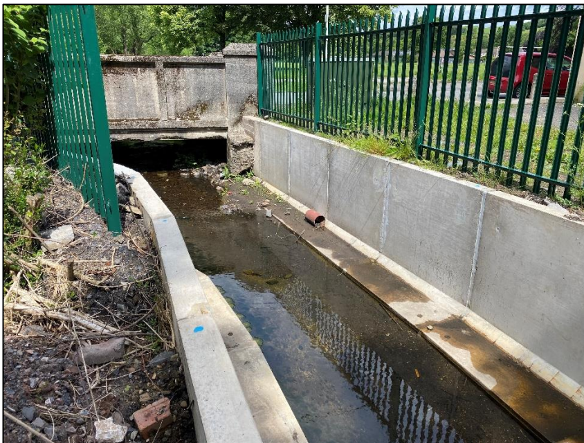
Photograph 6: Emerging concrete culvert southern side of the bridge.
