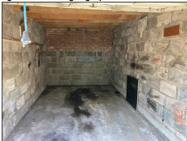
Figure 4 – Internal garage space
