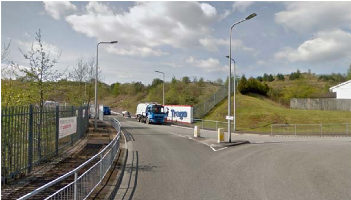
Plate 1 – view of PFS site from southeast
