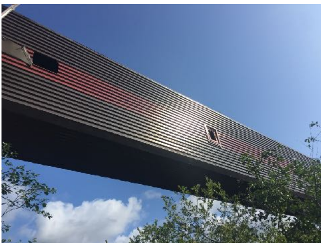
View of gantry over River Taff
