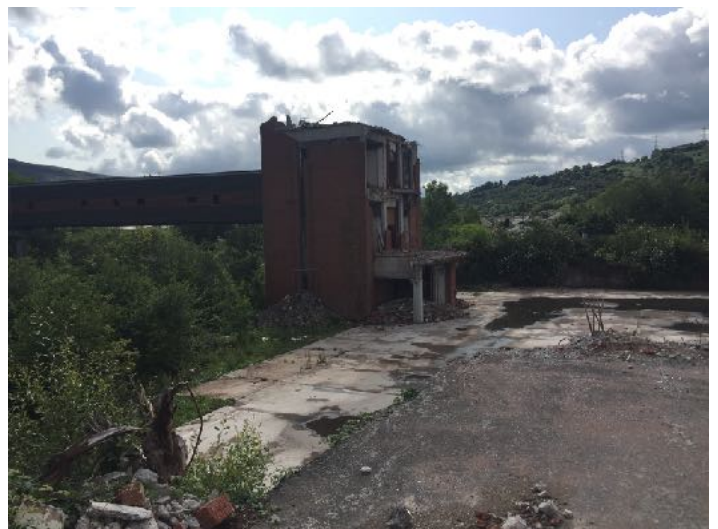
View of south east corner of site
