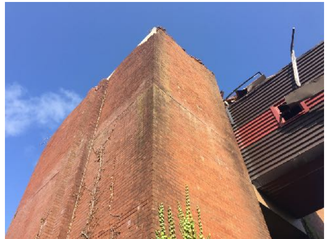
View of Office tower remaining
