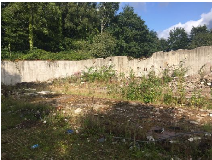
View of building foundations
