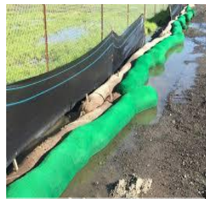
Fig.3.7 – Silt fence
