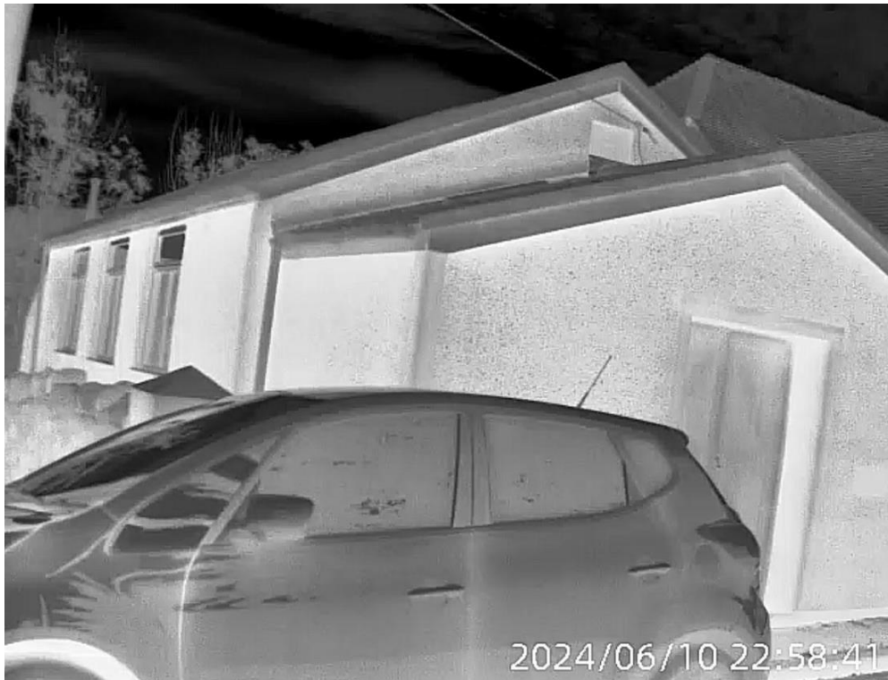
Figure 4- Thermal Guide camera view 10 th June 2024
