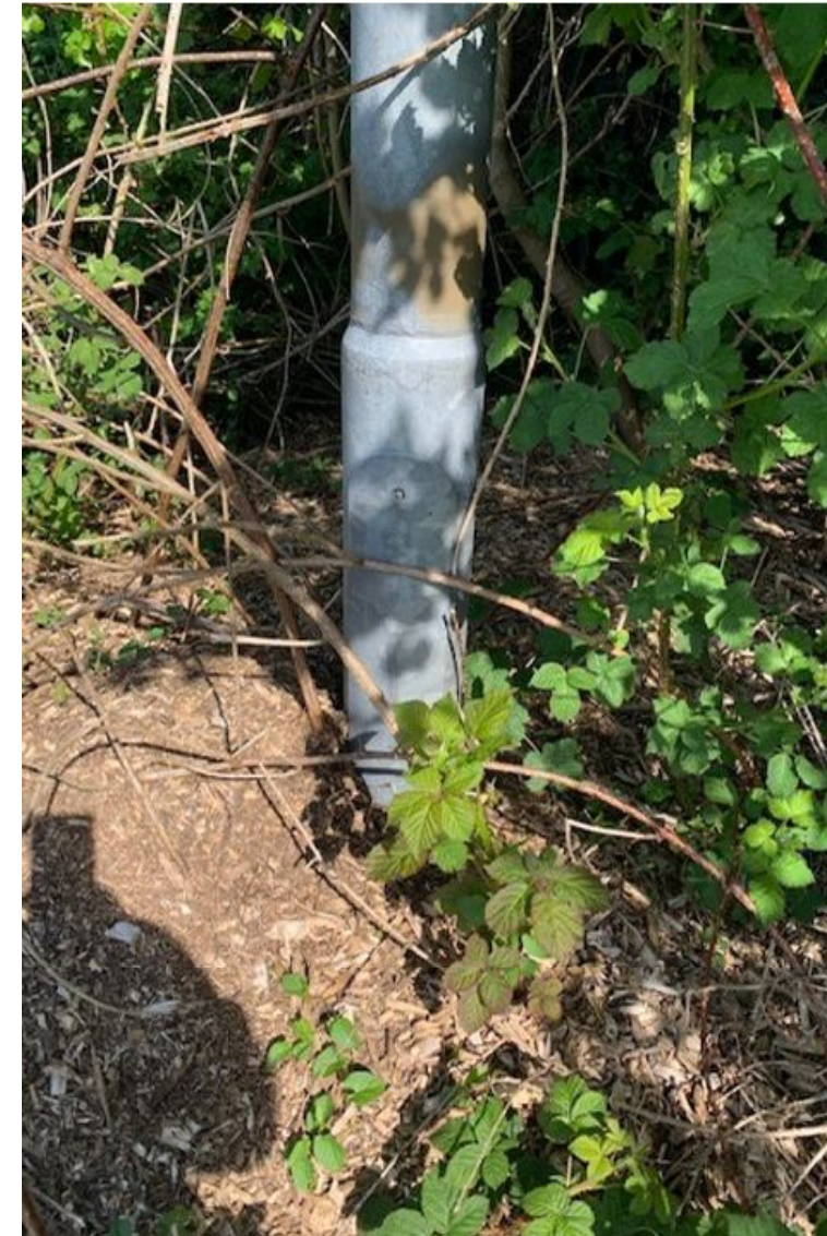
Existing Post 4 - base of post to be dug out to allow access into the cut out chamber
