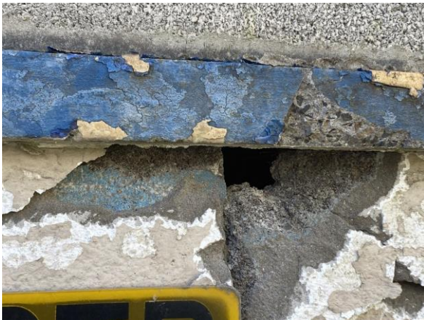
Photo 9: Cavity in External Wall Northern Front
