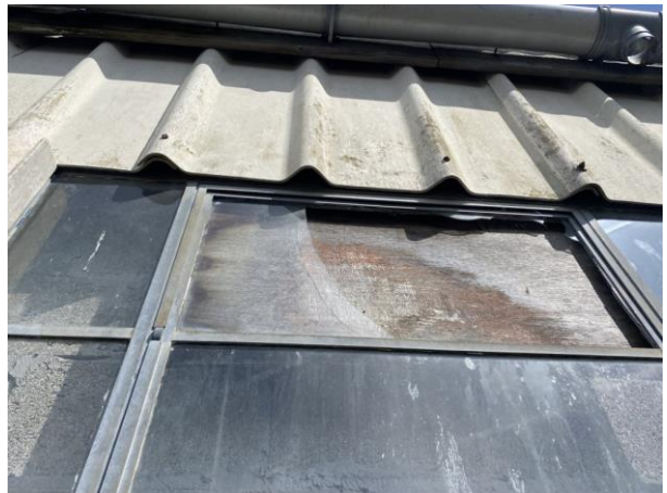
Photo 10: Southern Elevation Window Gaps
