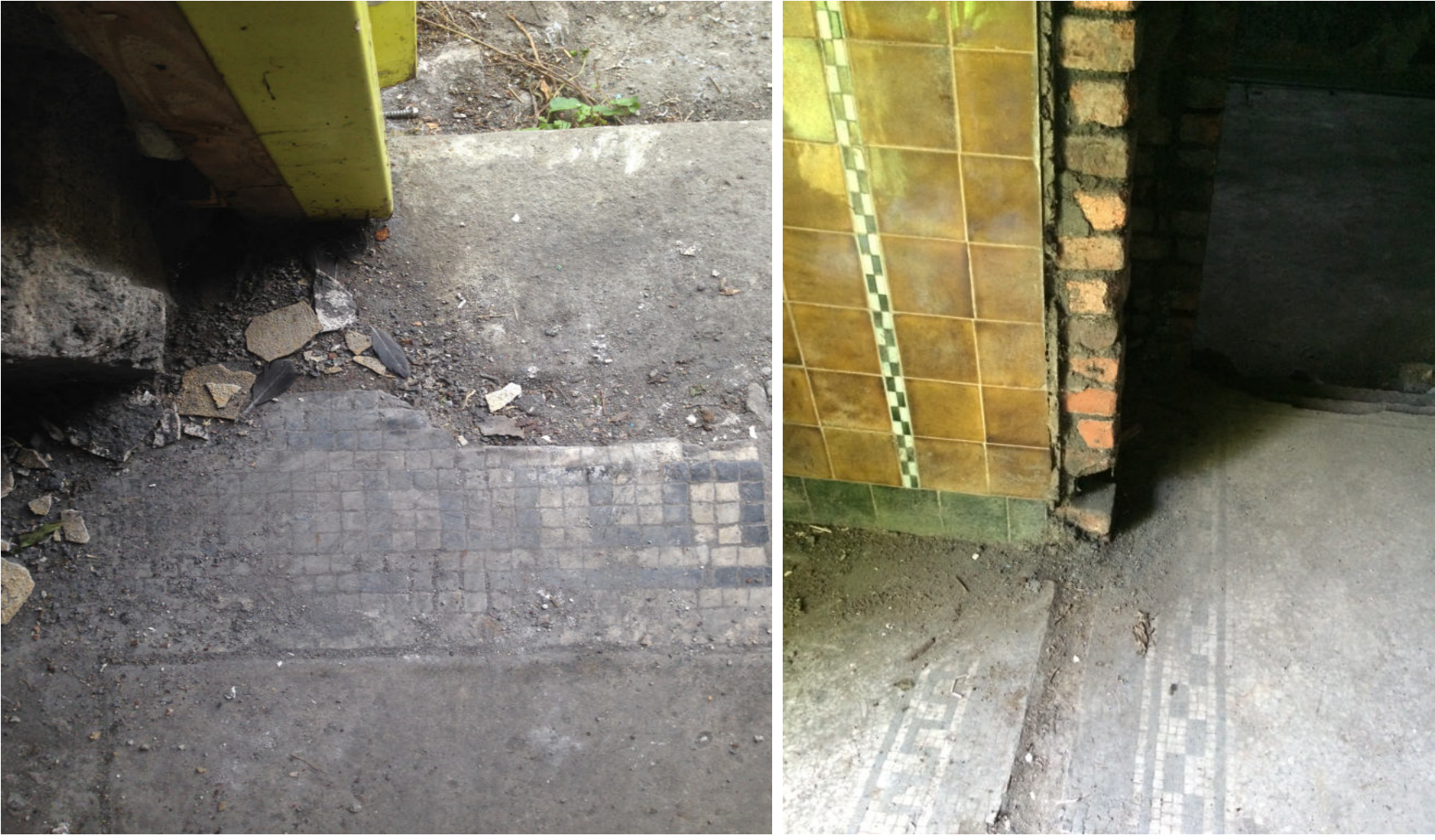
A 563.2 SITE PHOTOS EXISTING CONDITION
