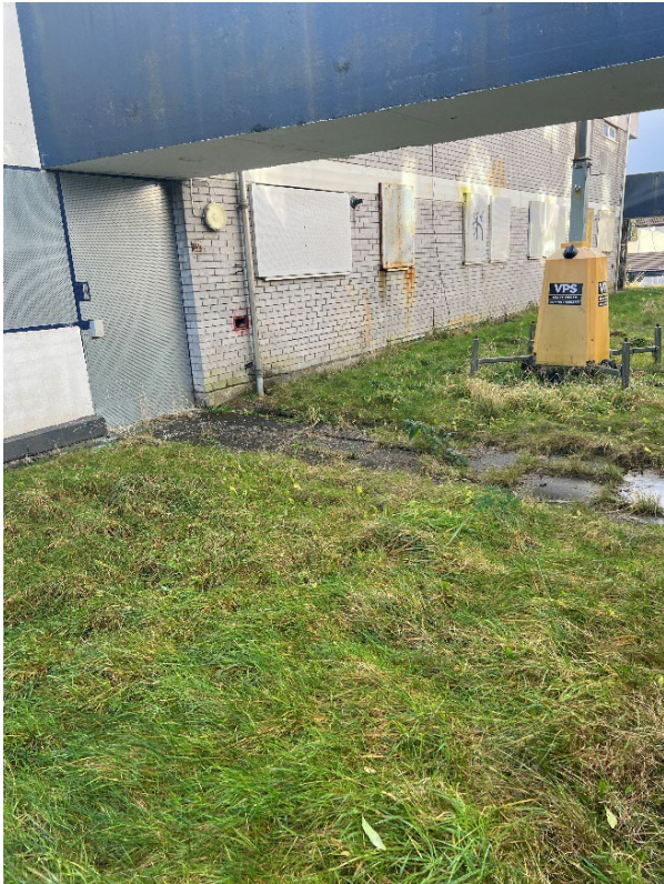
Grass area inside property
