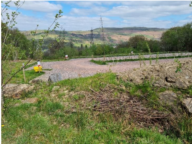
Figure 10 – View south across new car park area.
