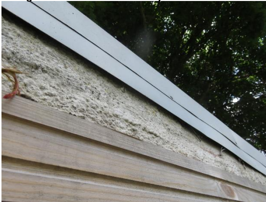
Plate 13: Gap beneath the barge board on the south facing elevation of the workshop
