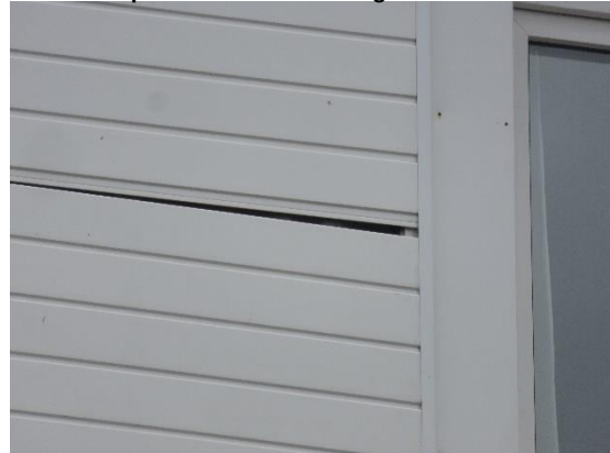
Plate 8: Gap in the uPVC cladding on the east side
