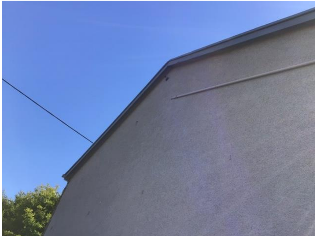
Figure 6 – Gable End of No48 High Street
