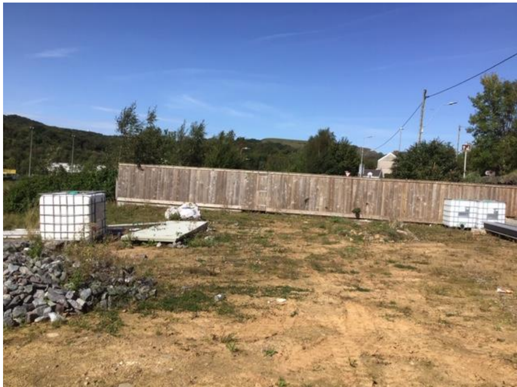
Figure 5: Site looking NW
